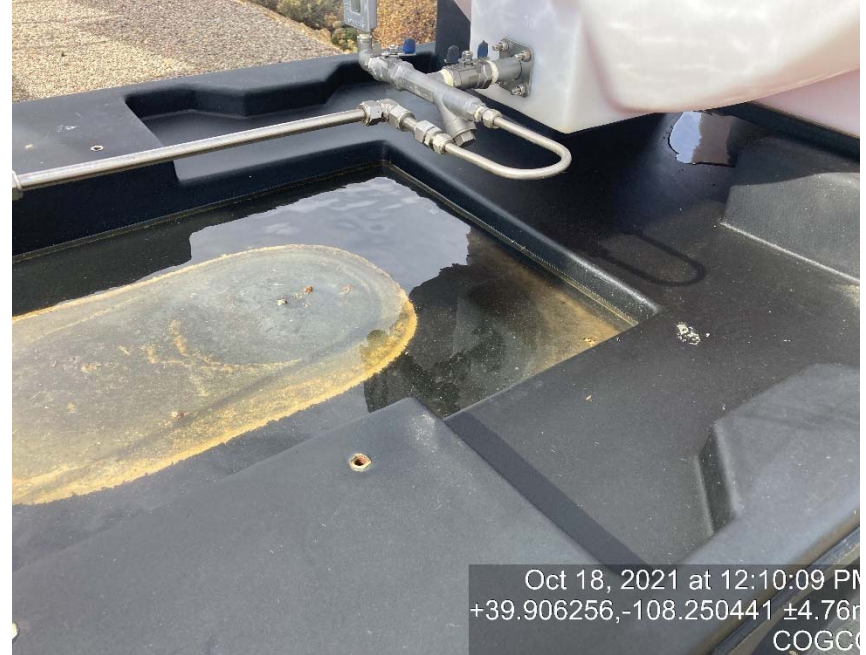
Chemical tank containment full of fluid
