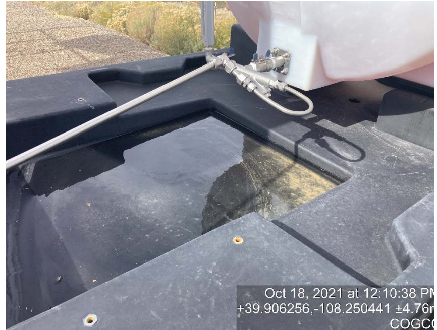
Chemical tank containment full of fluid
