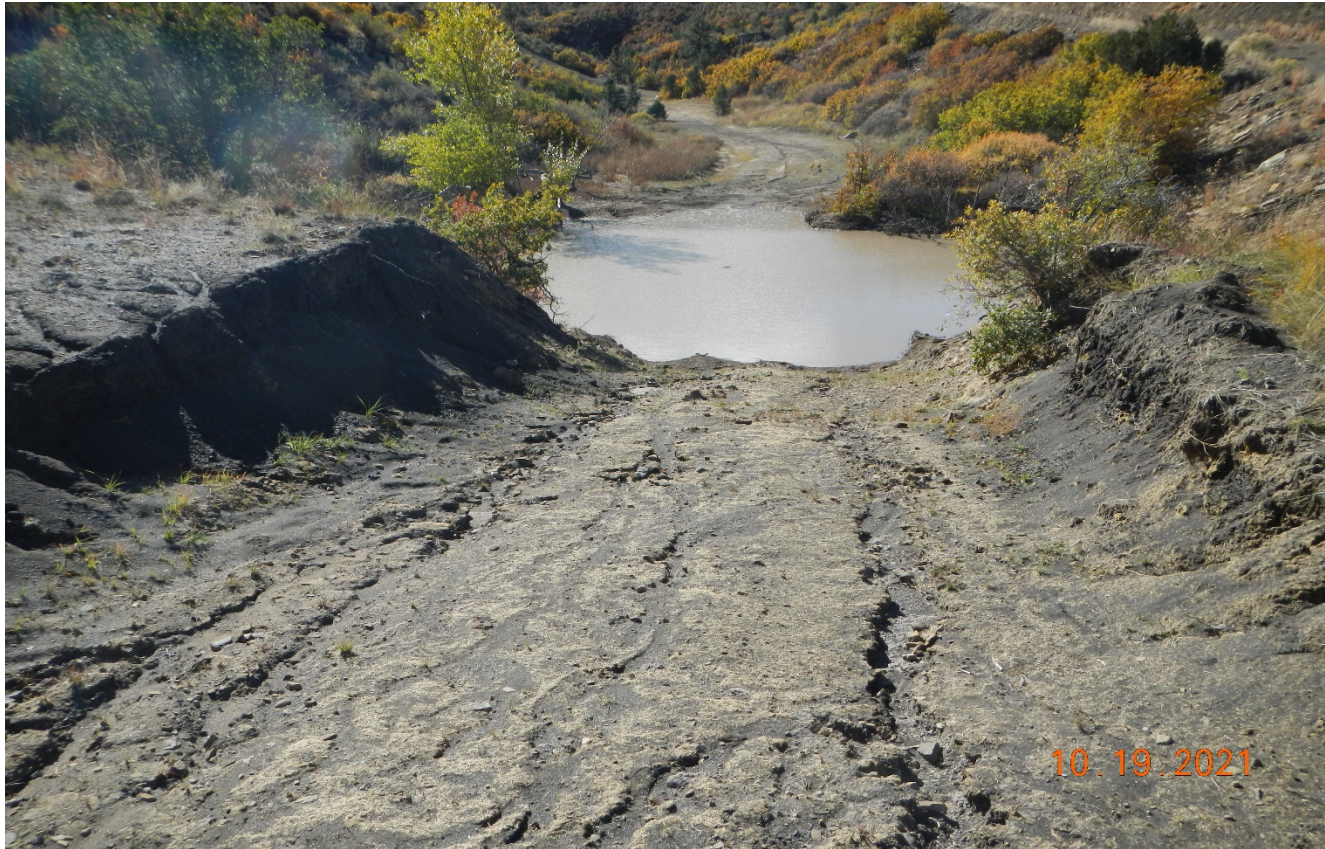
Photo 10. Facing south toward the road that was built to access the canyon bottom. There is erosion beginning to occur along this area which was not recontoured and reclaimed.
