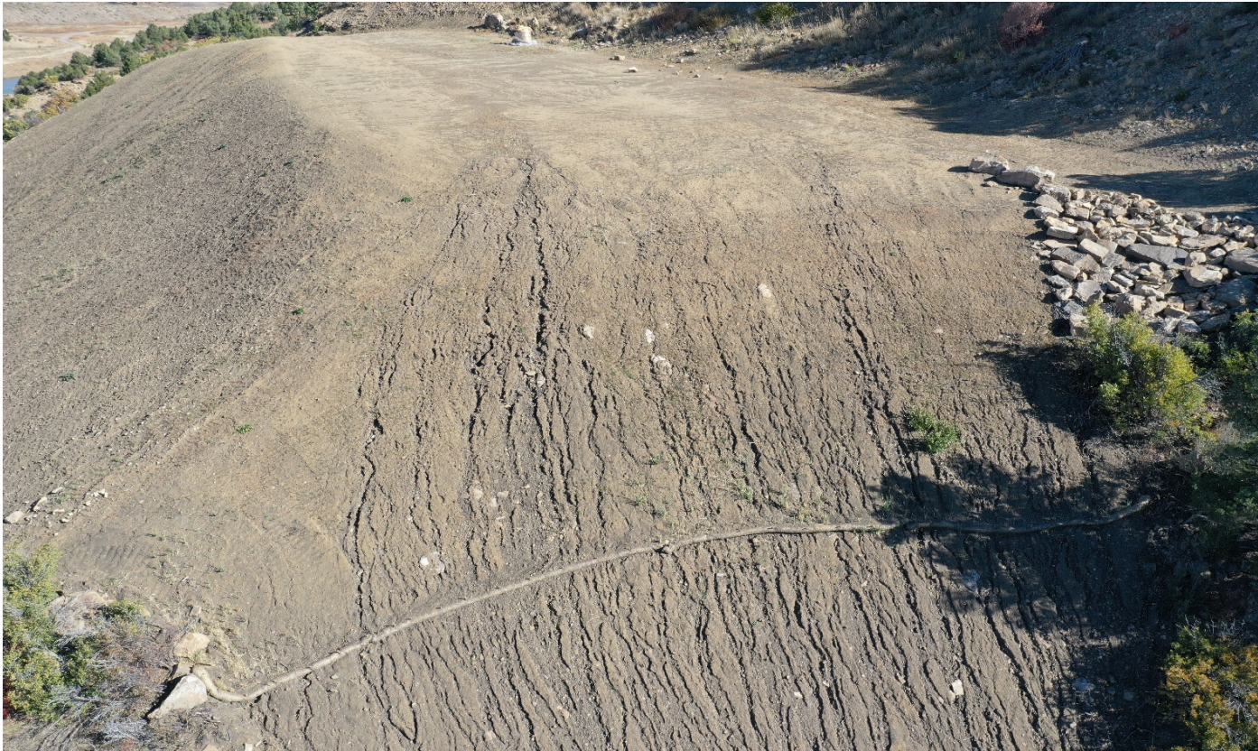
Photo 2. Facing north toward the location. There is now rilling erosion that occurred along the fill slope since the previous inspection. The stormwater BMP's are not sufficient as previously indicated and have not been maintained.
