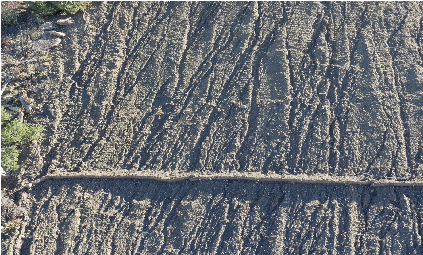
Photo 5. Facing closer to the fill slope shows the rilling erosion that has occurred. The wattles are not maintained and have filled in with sediment.
