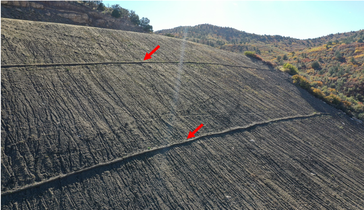
Photo 4. Facing east toward the fill slope. Stormwater controls were not sufficient and erosion has since occurred along the fill slope. The red arrows point to the two rows of wattles that are now filled in with sediment since previous inspection.
