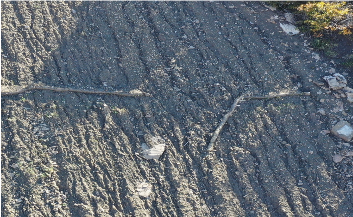
Photo 6. The straw wattles along the cut slope are displaced and not maintained. Previous corrective action was not performed.
