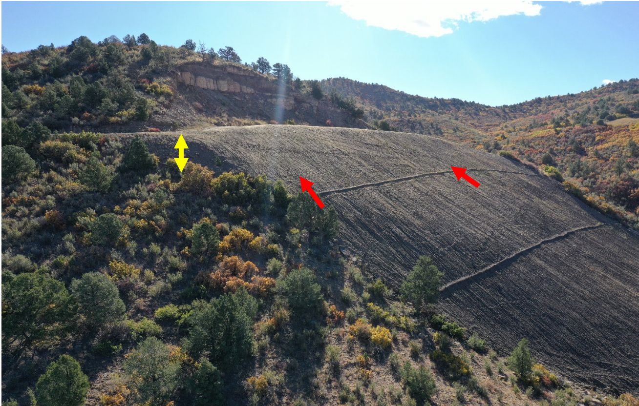
Photo 7. Facing east toward the location which was not recontoured per the rules. The red arrows point to fill material which could have been pushed back to original contour. The yellow arrow shows fill material which is about 20ft. from the original grade.
