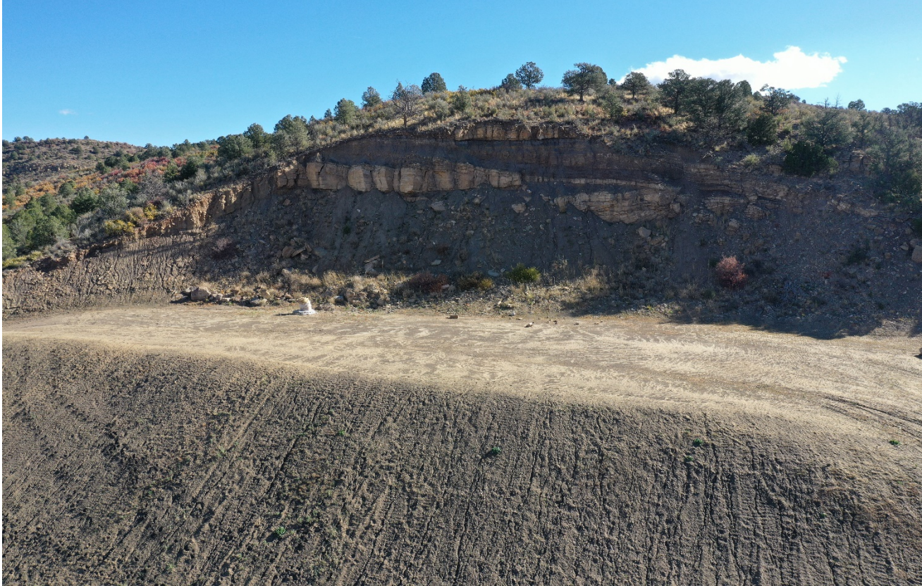
Photo 3. Facing northeast toward the location. A vertical unstable cut slope still remains. The fill slope material was not resloped back to the cut slope.
