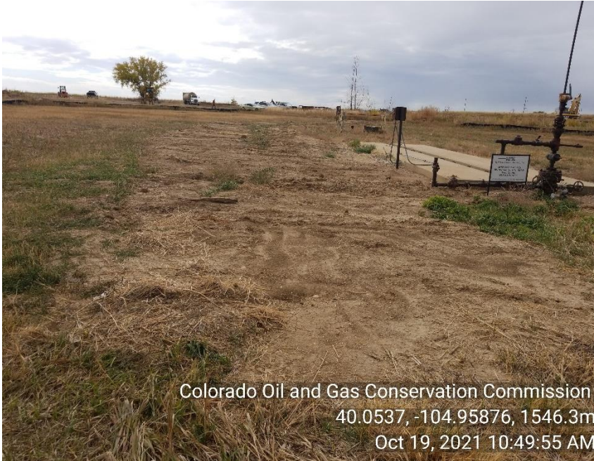
Photo 3 No BMP's in place along backfilled ditch. Area is not seeded or graded.
