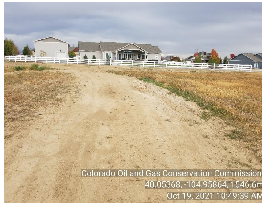
Photo 2 access road has deep ruts no BMP's in place or maintenance performed.
