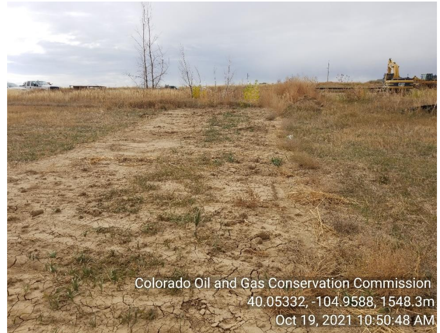
Photo 6 No BMP's in place on backfilled ditch.
