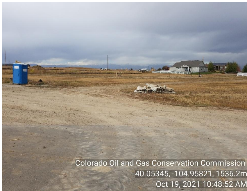
Photo 1 not tracking pad onto asphalt.
