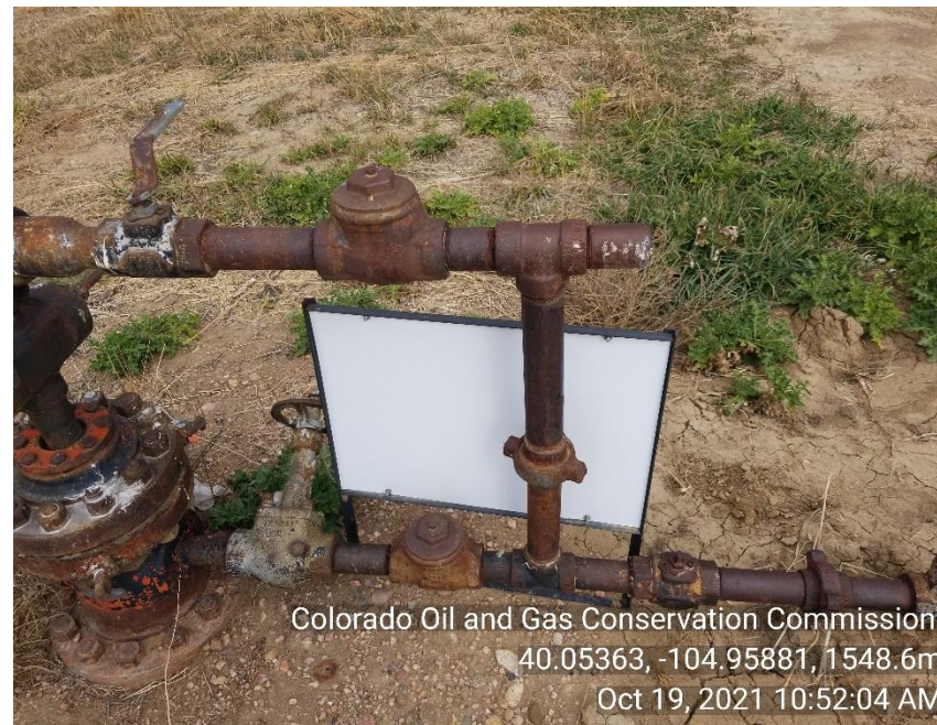
Photo 8 Well head flow line valves is the closed position.
