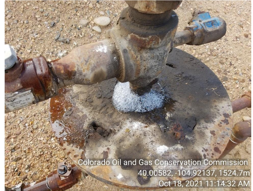
Photo 4 Mechanical issue well head leaking.
