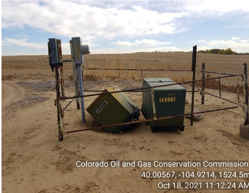
Photo 3 Mechanical issue electric panel sinking and wires showing
