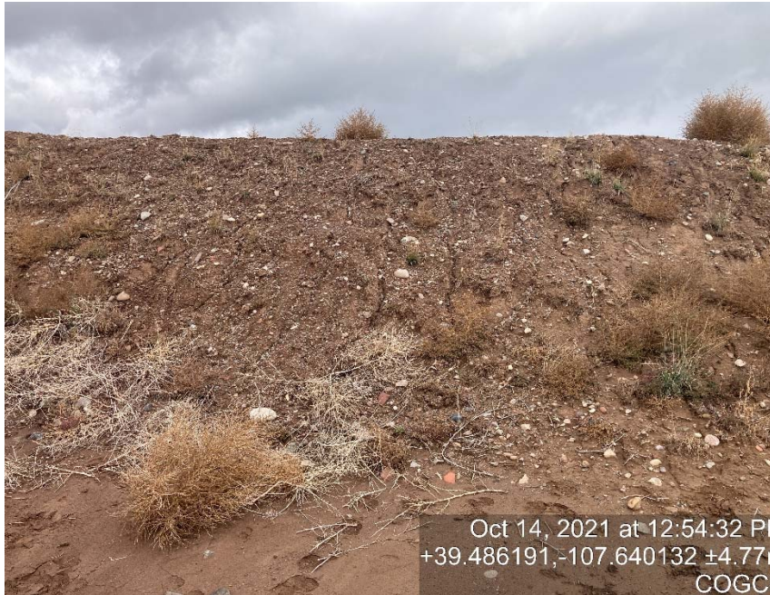
Lack of stabilization/erosion
