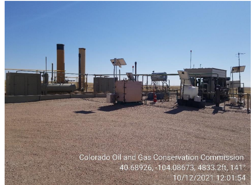
Photo 6 – Compressor, VRU and Separators
