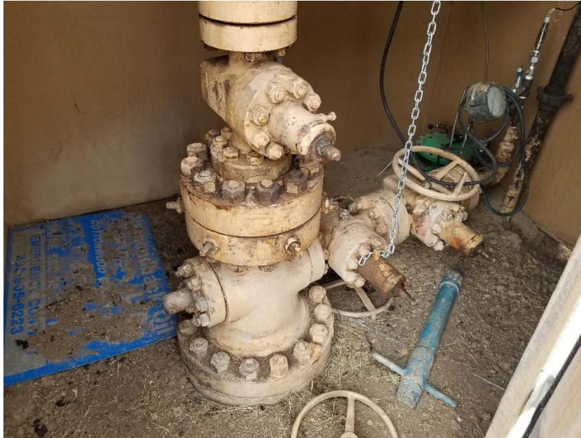
Photo 2. No bradenhead access apparent.
