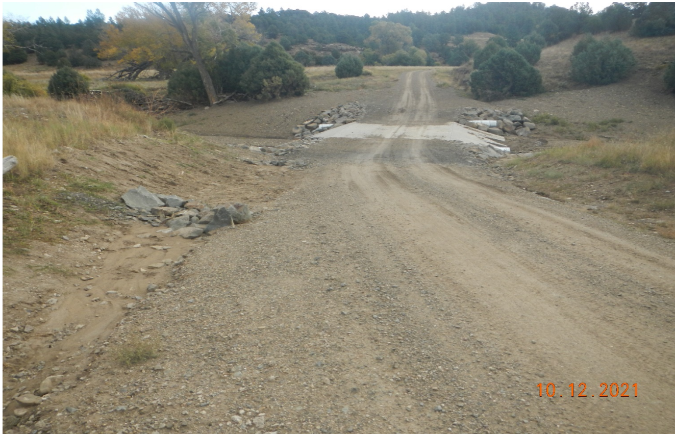
Photo 1. Facing east toward the access road stream crossing. The road side area was repaired and rock check dams were installed.
