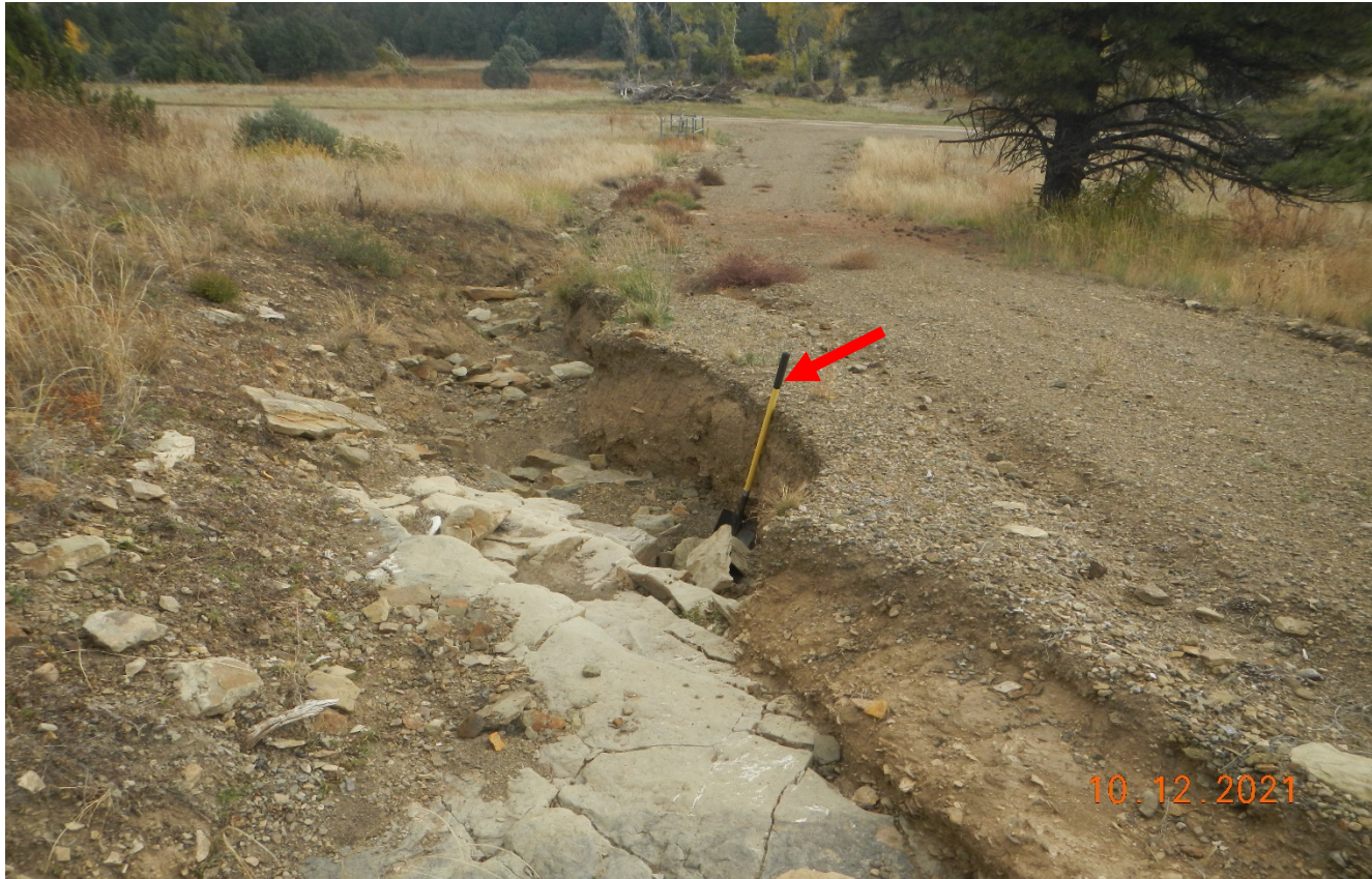
Photo 4. Facing back down the road. The erosion along the road side has not been repaired and stabilized. Arrow points to 4.5 ft. shovel.
