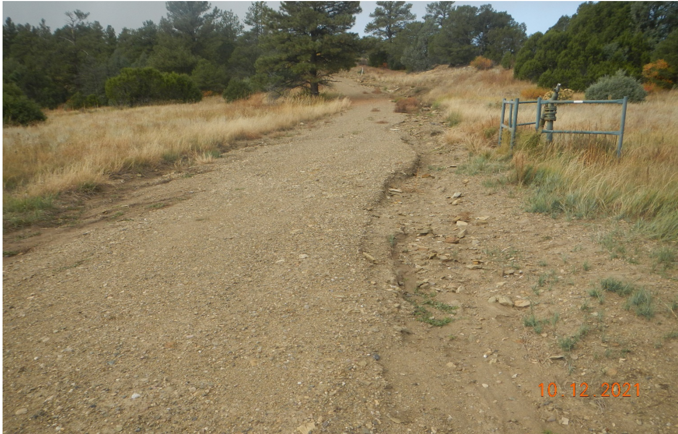
Photo 3. Facing southwest toward the access road. This area of erosion has not been repaired and stabilized. Previous corrective action was not completed.
