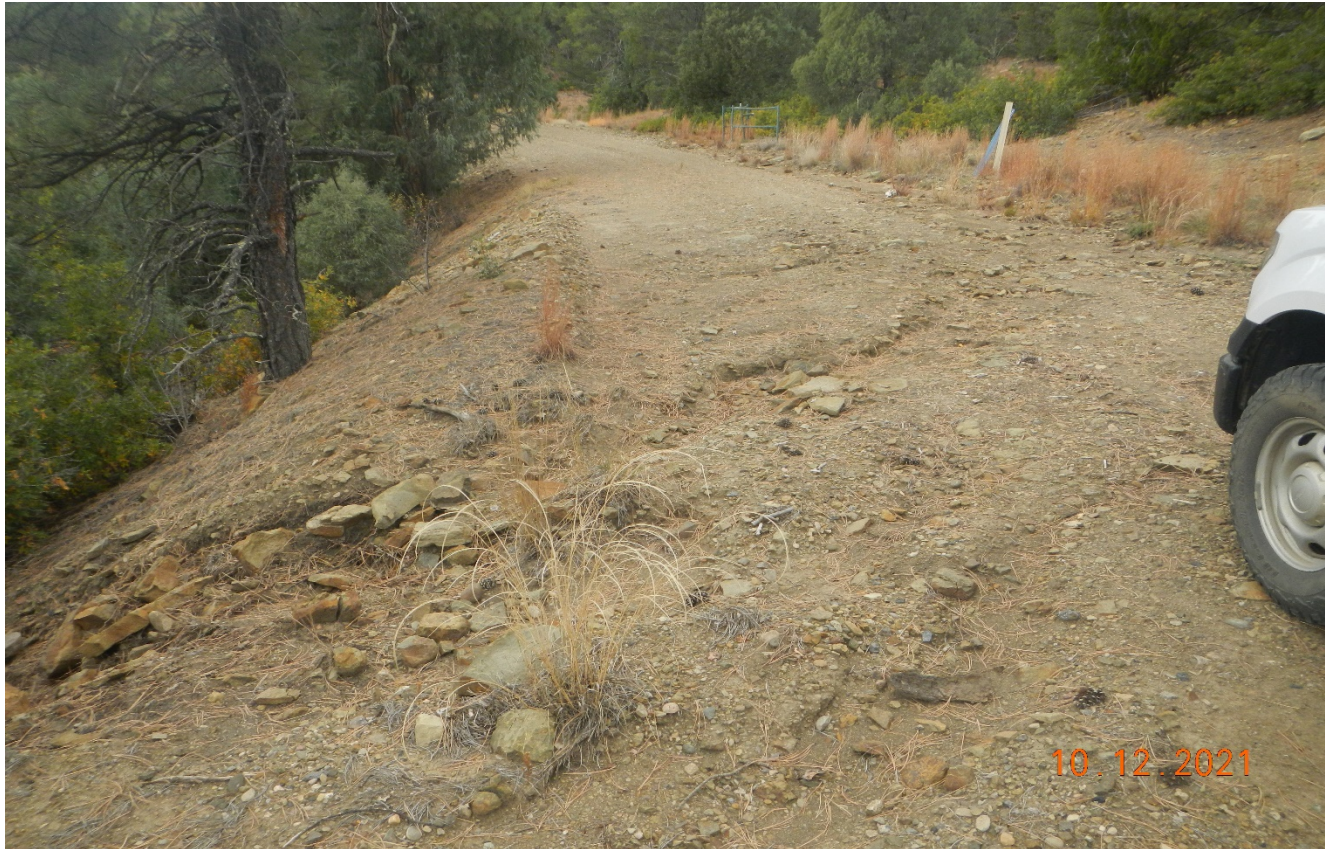
Photo 5. Further up the access road. There is stormwater erosion across the road. This area may need a culvert.
