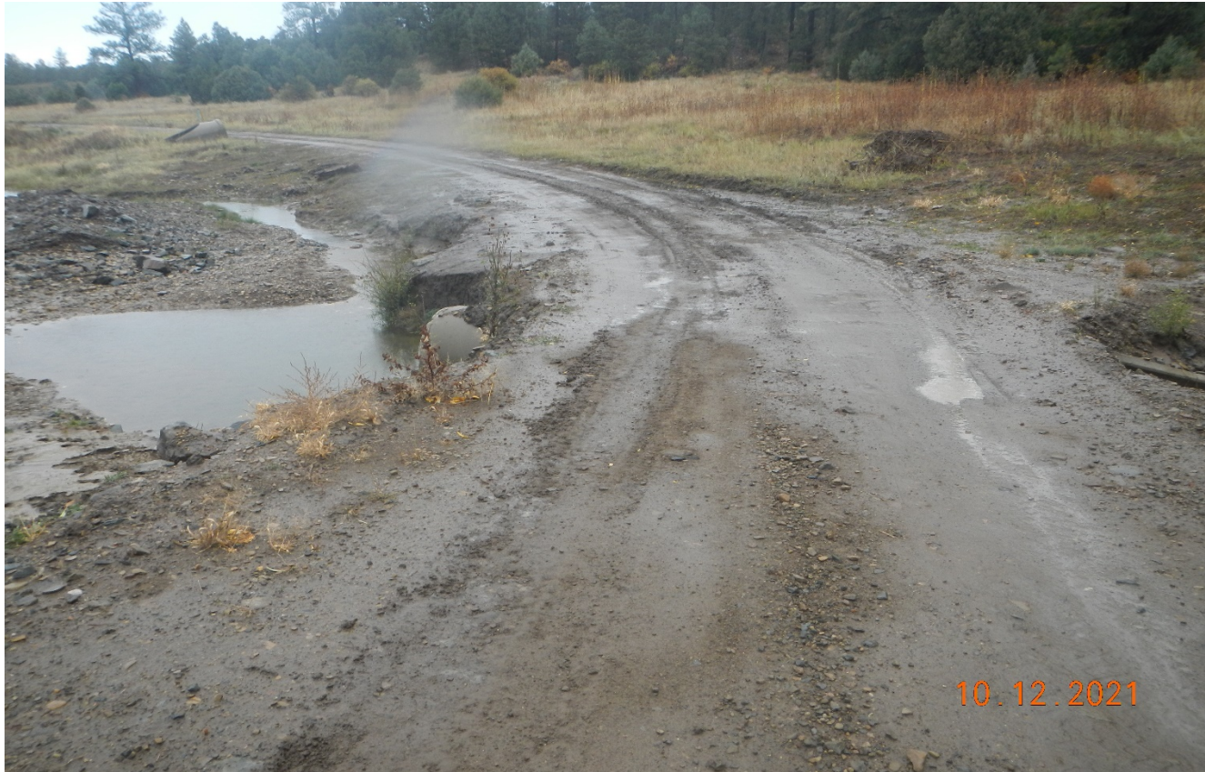
Photo 6. Facing back to the northeast at the stream crossing further along the road. This area of the road needs to be stabilized with gravel as well as bank stabilization.
