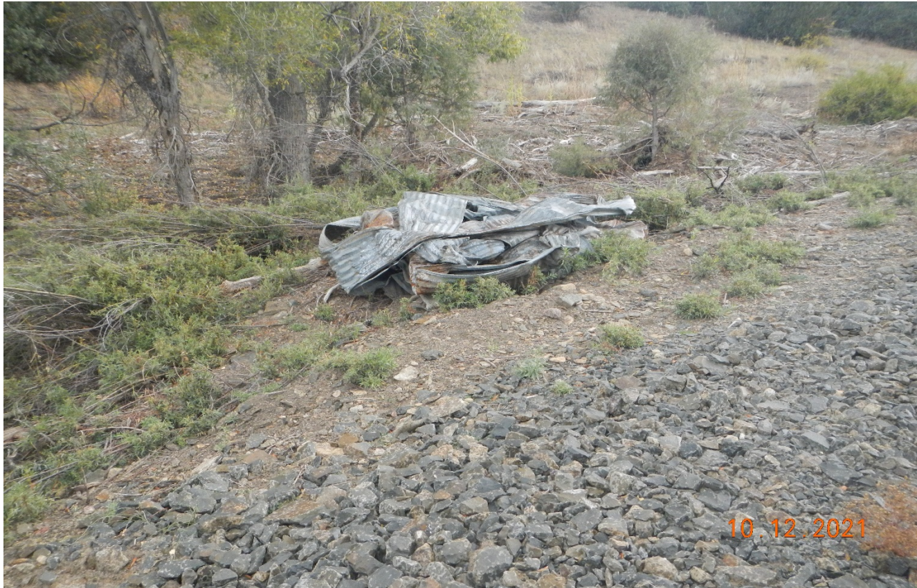
Photo 2. The damaged culverts need to be removed.
