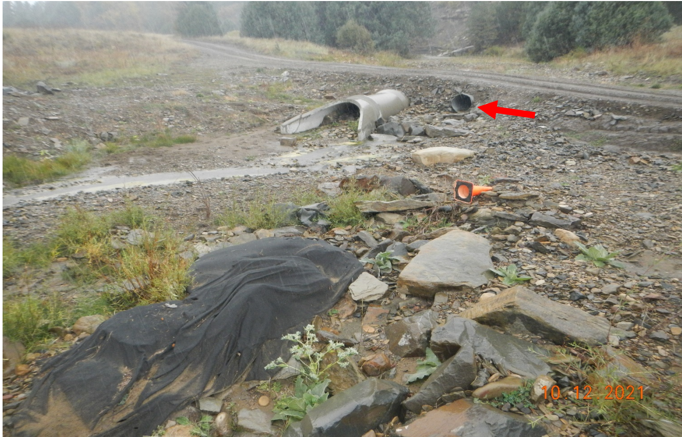
Photo 5. The cement culvert is filled in with sediment. The culvert at red arrow is not sufficient as shown by the size of the previous culvert. The liner debris in lower portion of photo needs to be removed.
