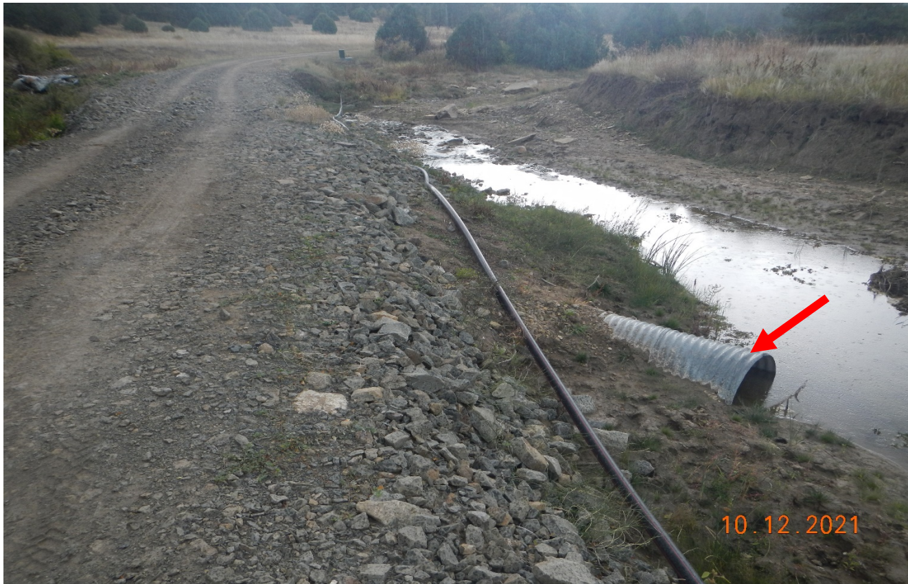
Photo 1. Facing southeast along the main access road. The black poly line remains exposed to potential damage. The culvert shown at red arrow is filled in with sediment on the opposite side.
