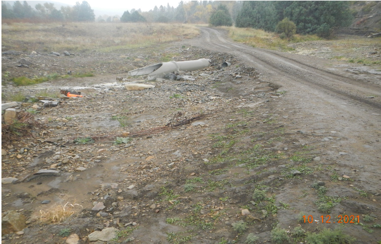
Photo 3. Facing southwest along the main road. There is a culvert installed for temporary passage. An engineered size culvert will be needed along with bank and inlet/outlet protection. Previous corrective action was not completed.
