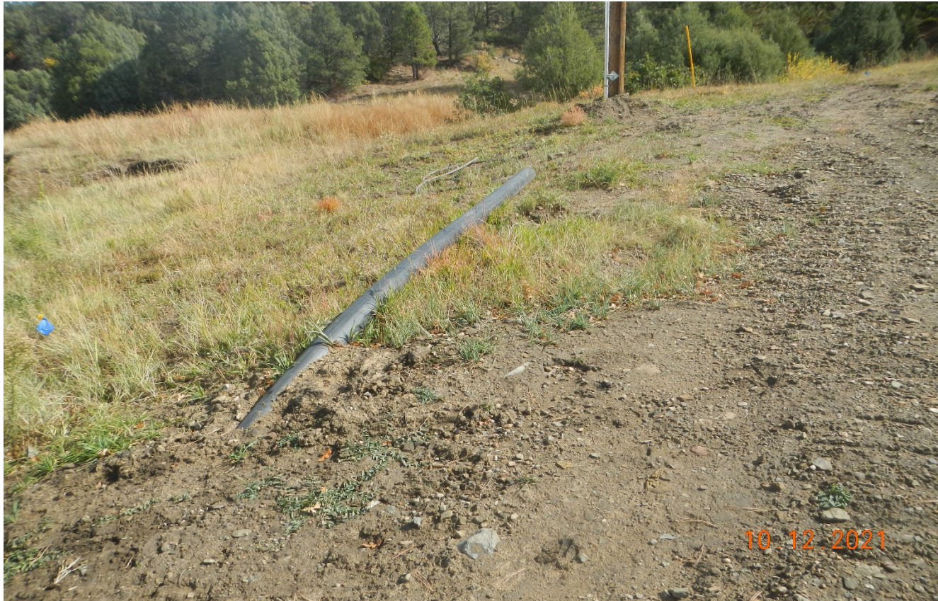
Photo 4. There is a black plastic pipe extending out of the ground on the east side of stream crossing. This needs to be removed or repaired.
