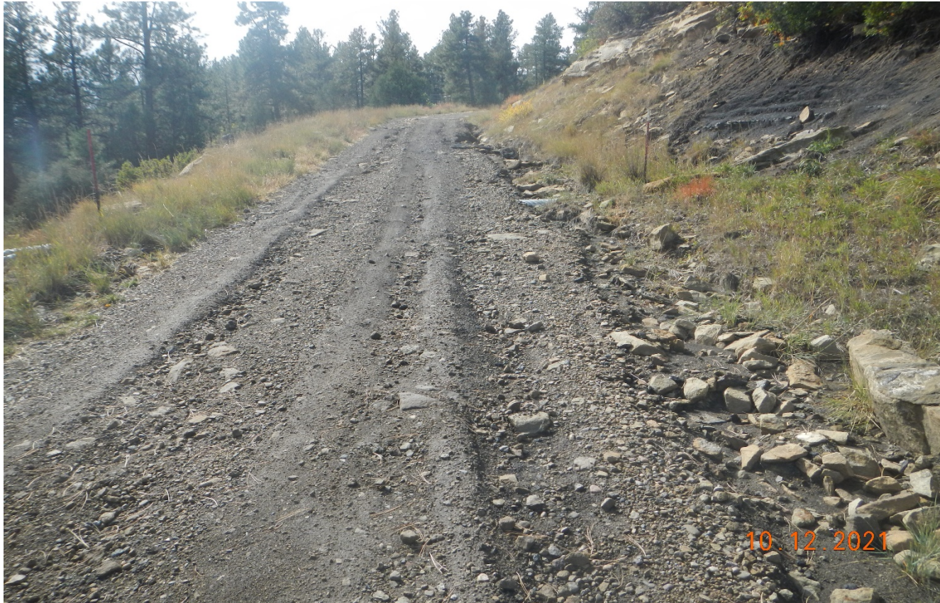
Photo 6. The culverts along the access road are filled in with sediment causing stormwater erosion down the road.
