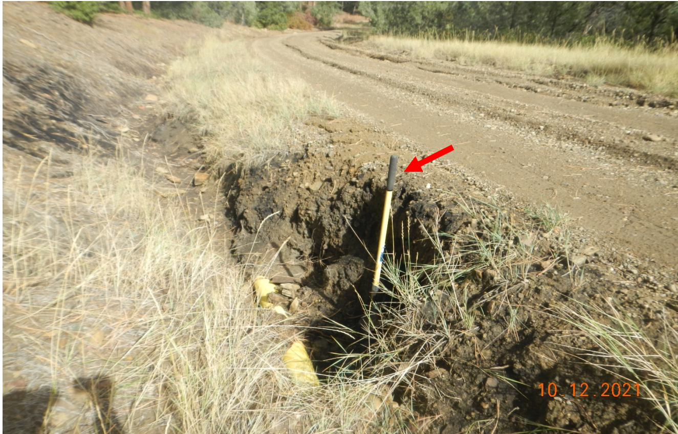
Photo 9. Erosion along the roadside has exposed a pipeline. Arrow points to 4.5 ft. shovel.
