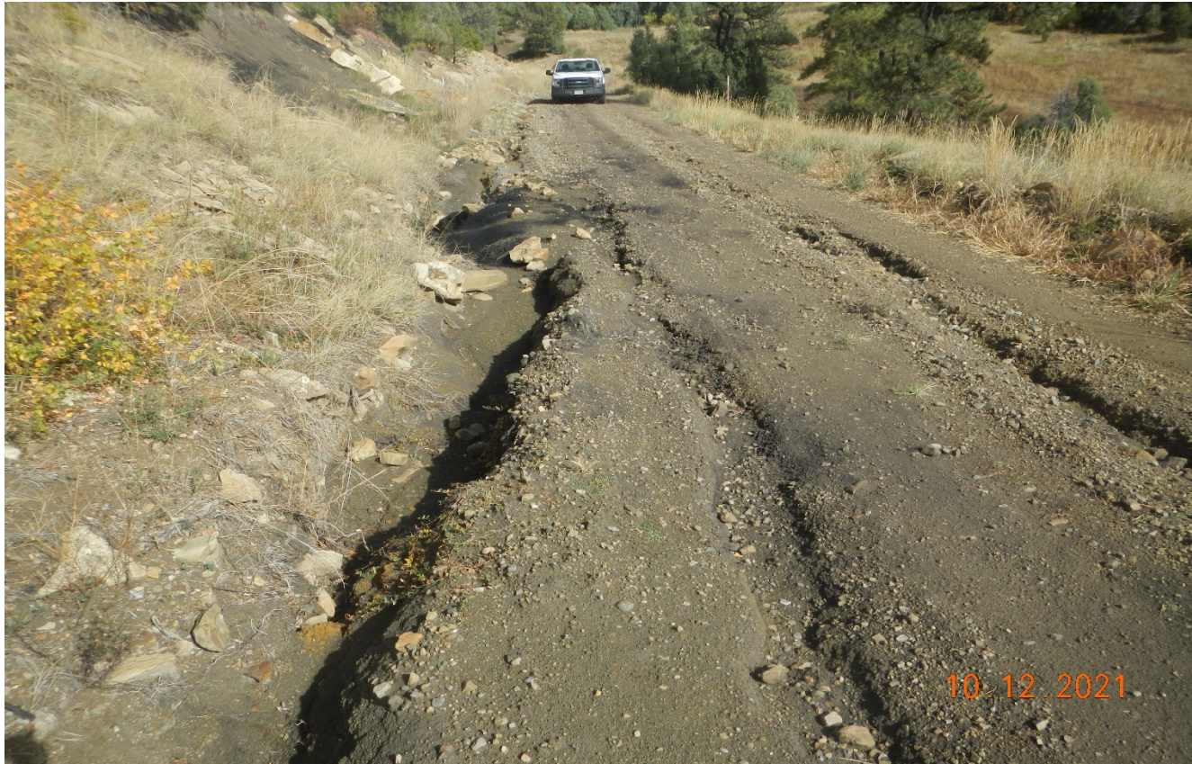
Photo 7. Facing back down the road. There is erosion along the road side and stormwater is bypassing culverts which will cause further erosion. BMP's need to be repaired.
