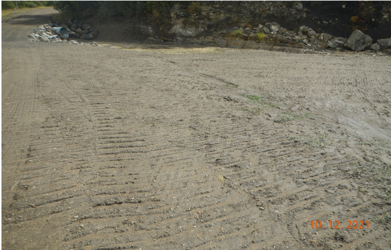
Photo 2. Facing toward the disturbance area along the road side. All disturbed areas along the road side need to be seeded and stabilized.
