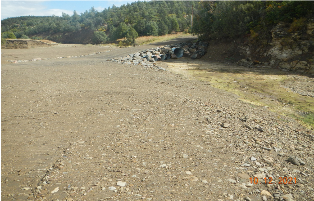
Photo 3. There are multiple culverts installed and rock rip/rap was installed for bank stabilization.
