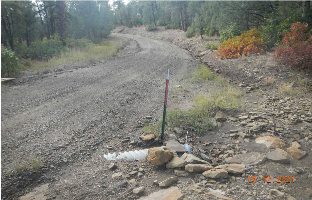
Photo 8. Another culvert further along the road is filled in with sediment.
