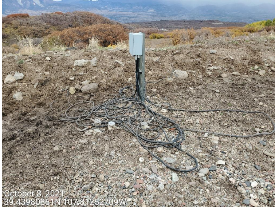
Photo 1: Photos shows electrical box and wires observed on the north end of the Location; wires observed to be disconnected, exposed and laying on the surface; equipment is unused.
