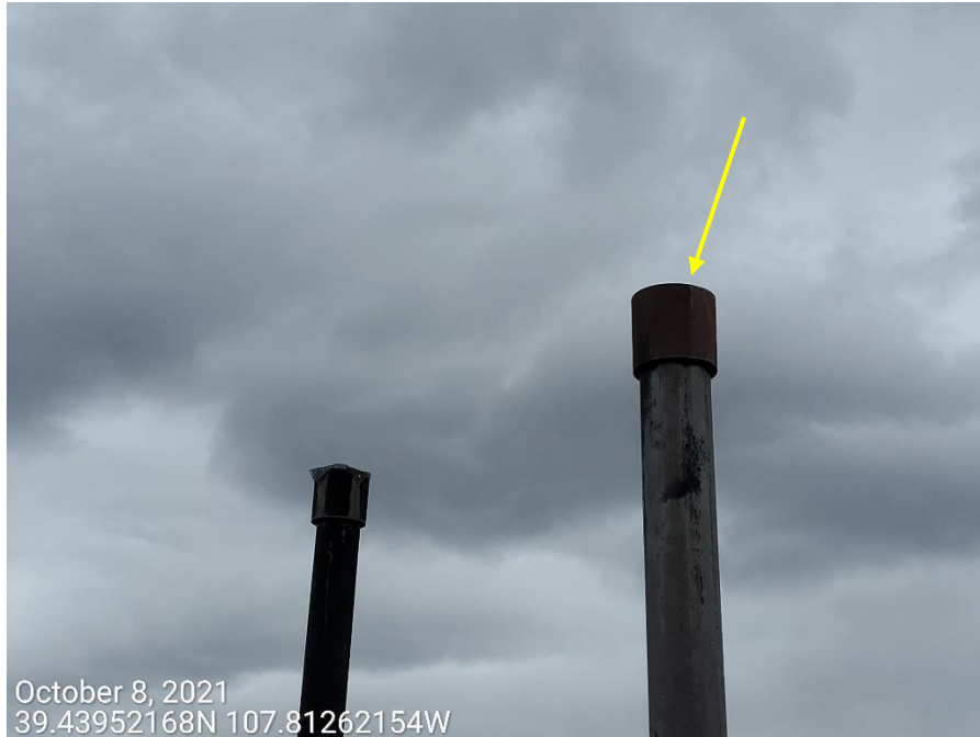
Photo 2: Photos taken from the separator equipment. Photos show wildlife protection screen has been installed on the northern separator, however, screen was not observed on the southern separator (arrow)
