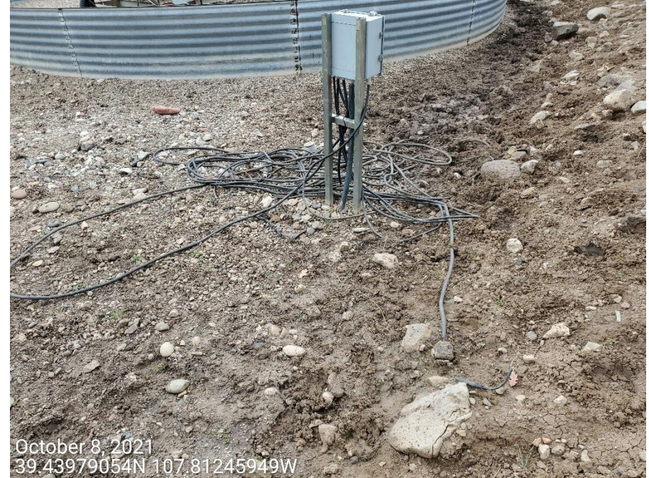
Photo 1: Photos shows electrical box and wires observed on the north end of the Location; wires observed to be disconnected, exposed and laying on the surface; equipment is unused.
