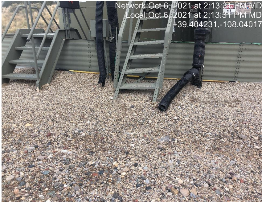
Photo #5031 Flowline heating insulation open ended and not capped.
