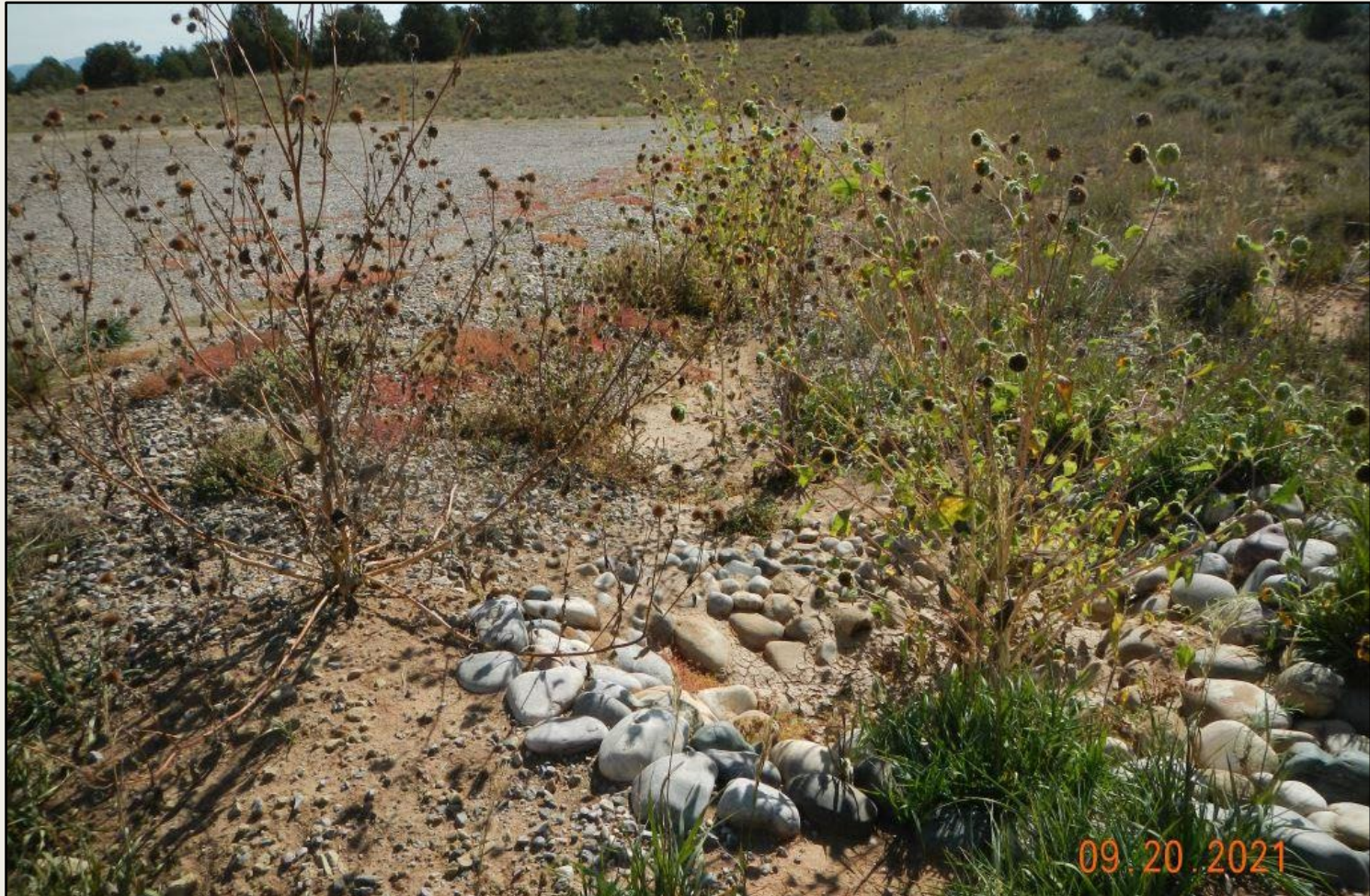
Photo 4. View of silt trap in the southwestern corner of the project area. This BMP is not adequate to contain diverted stormwater flows from the well pad, as evidenced by active down-slope erosion (Photo 3).
