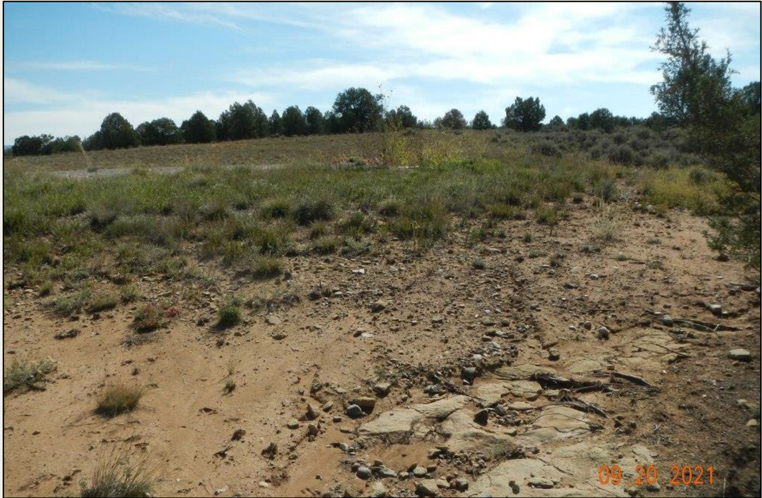
Photo 3. Another view of erosion occurring along the edge of the western project area. Diverted stormwater flows are scouring soils and vegetation in the southwestern corner.
