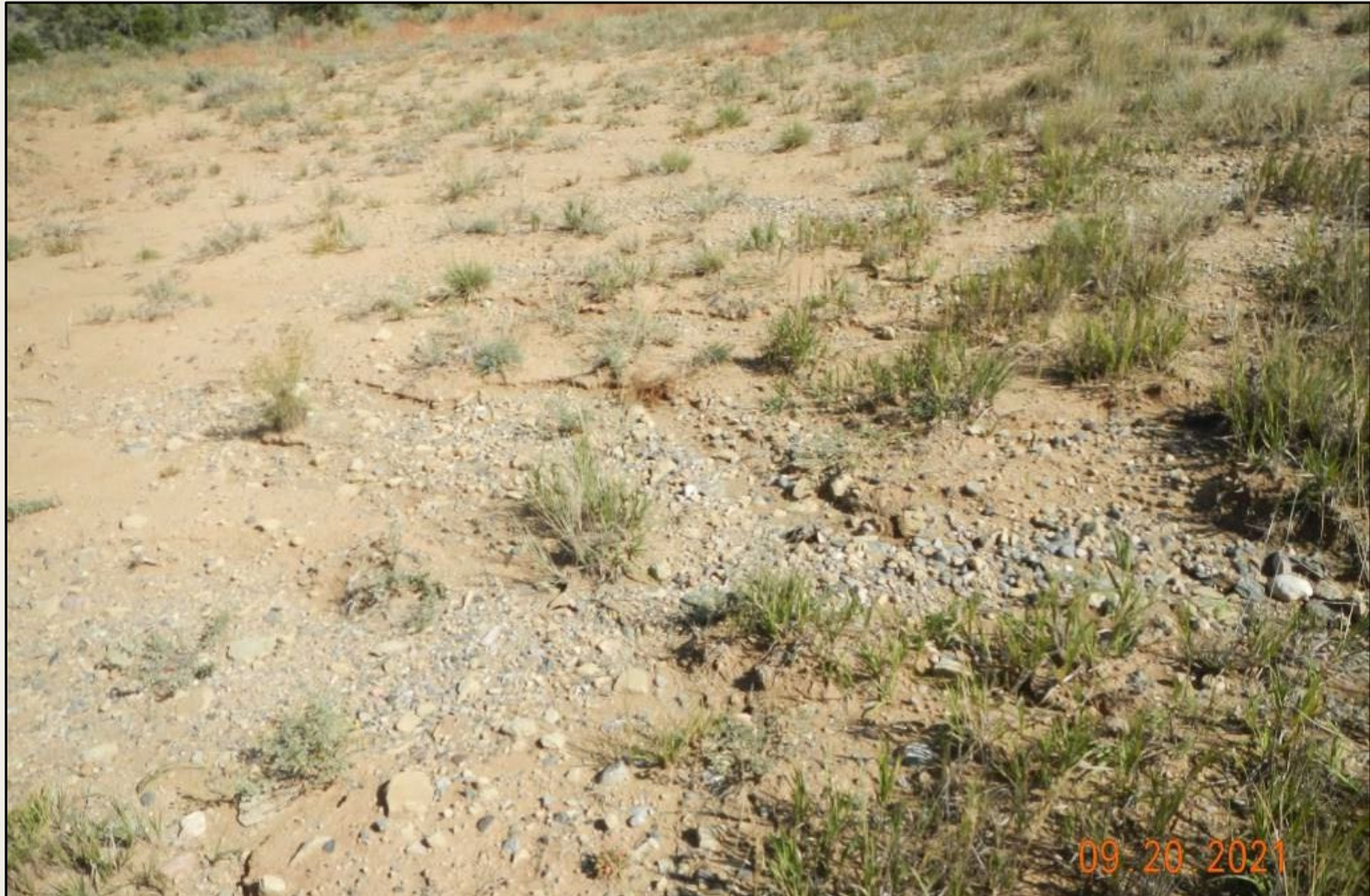
Photo 2. View of western fill slope. Revegetation is progressing with western wheatgrass, smooth brome, and crested wheatgrass. Erosion is occurring along the edges of the seeded area, at the toe of the slope.
