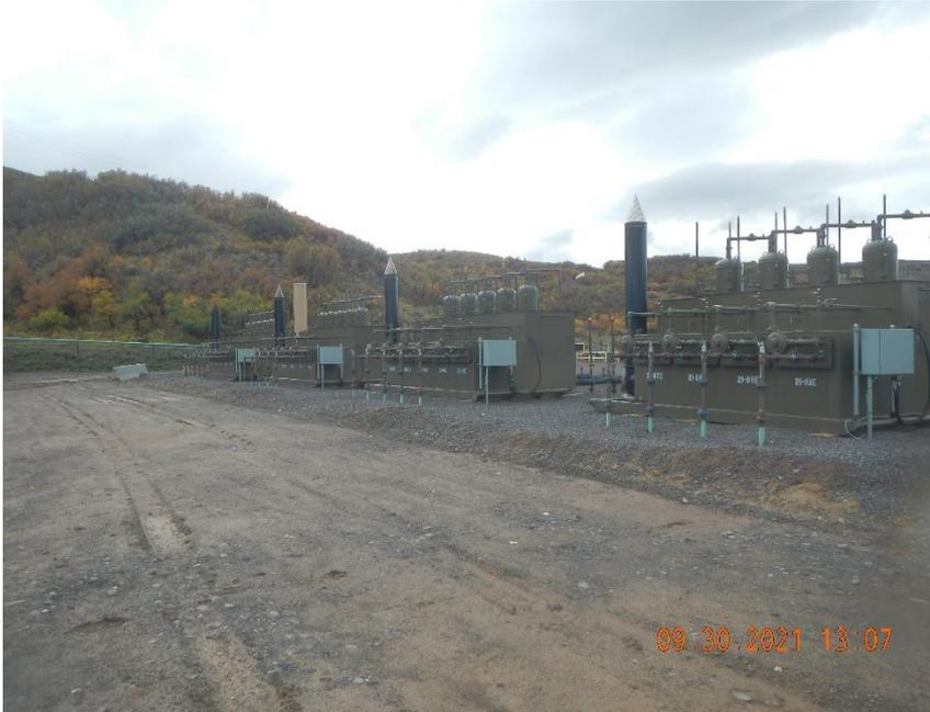
**Glycol storage vessels on heated separators have no labels.**
