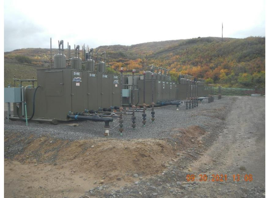
**Glycol storage vessels on heated separators have no labels.**
