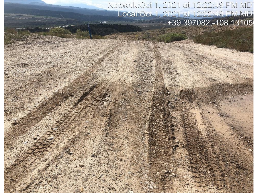
Photo #4999 No form of tracking BMP located at the entrance to location.
