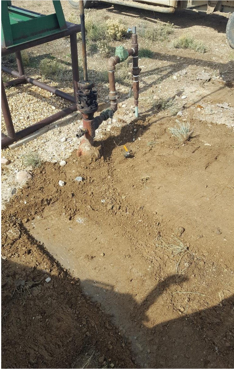
Figure #1 Bradenhead access has been installed.
