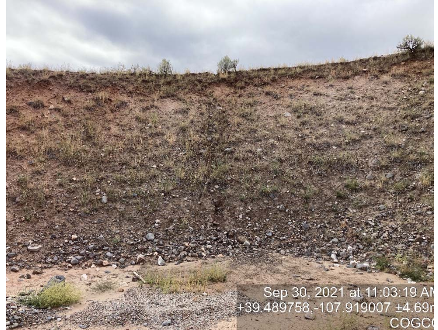
Lack of stabilization/erosion
