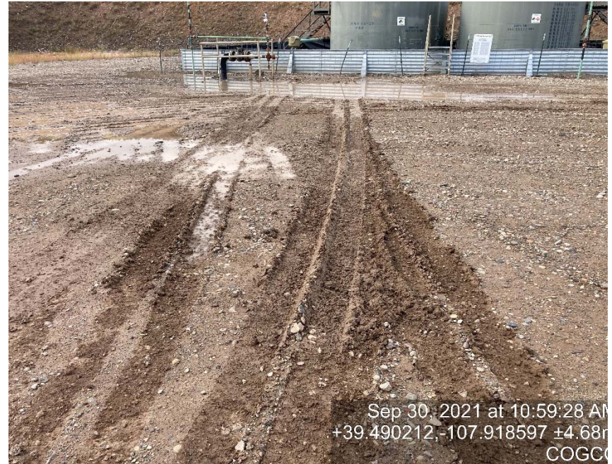
Lack of stabilization/compaction
