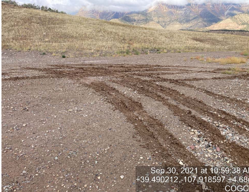
Lack of stabilization/compaction
