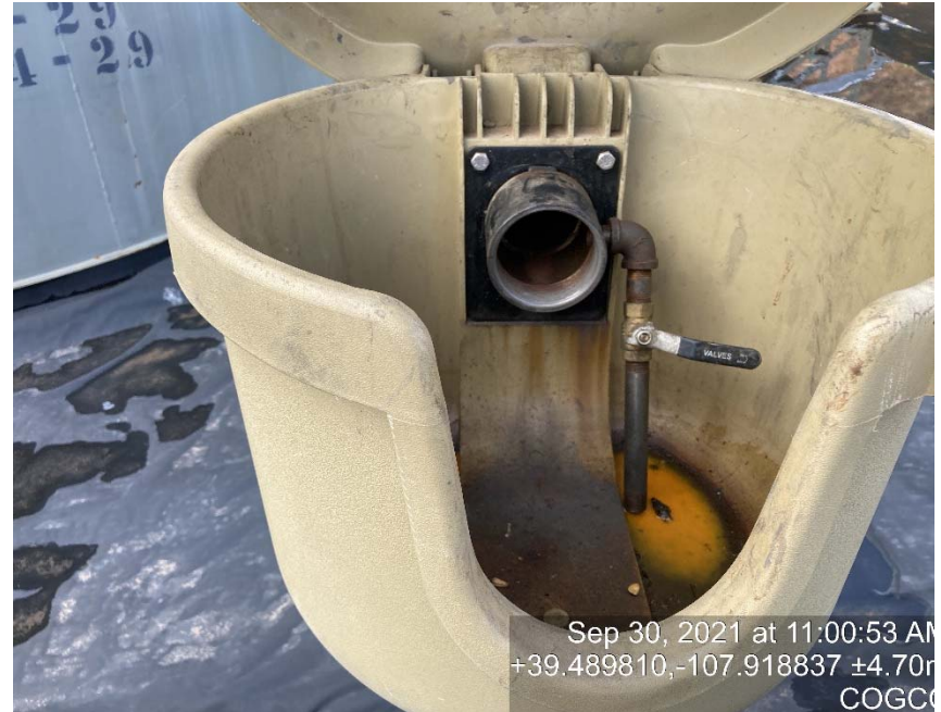
Missing bull plugs/caps on load out lines
