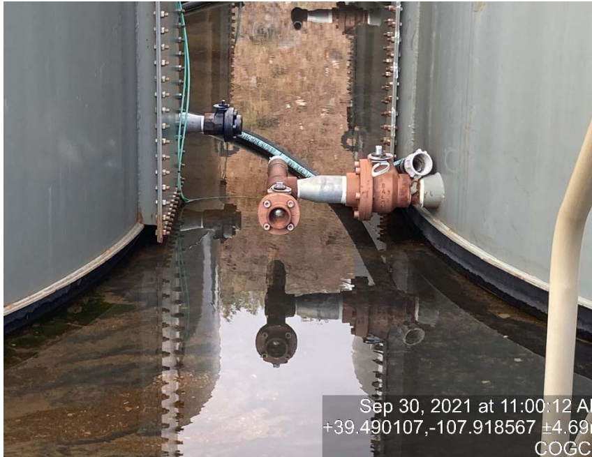
Missing bull plugs/caps on load out lines
