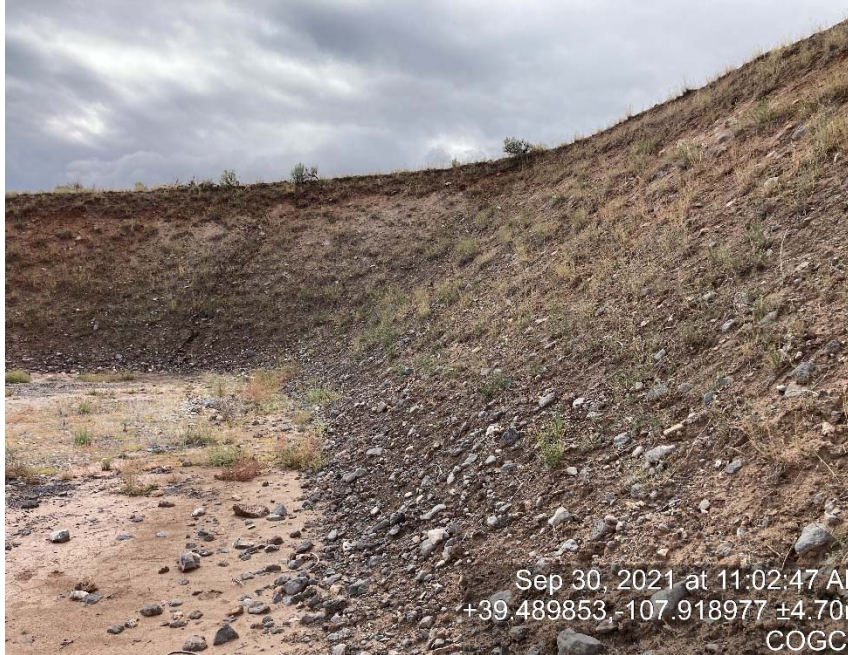
Lack of stabilization/erosion
