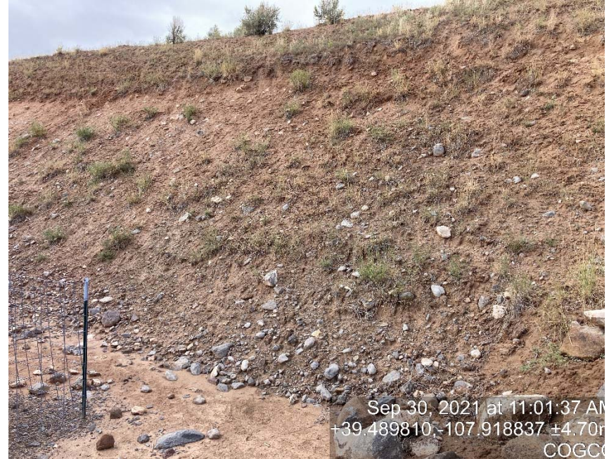
Lack of stabilization/erosion
