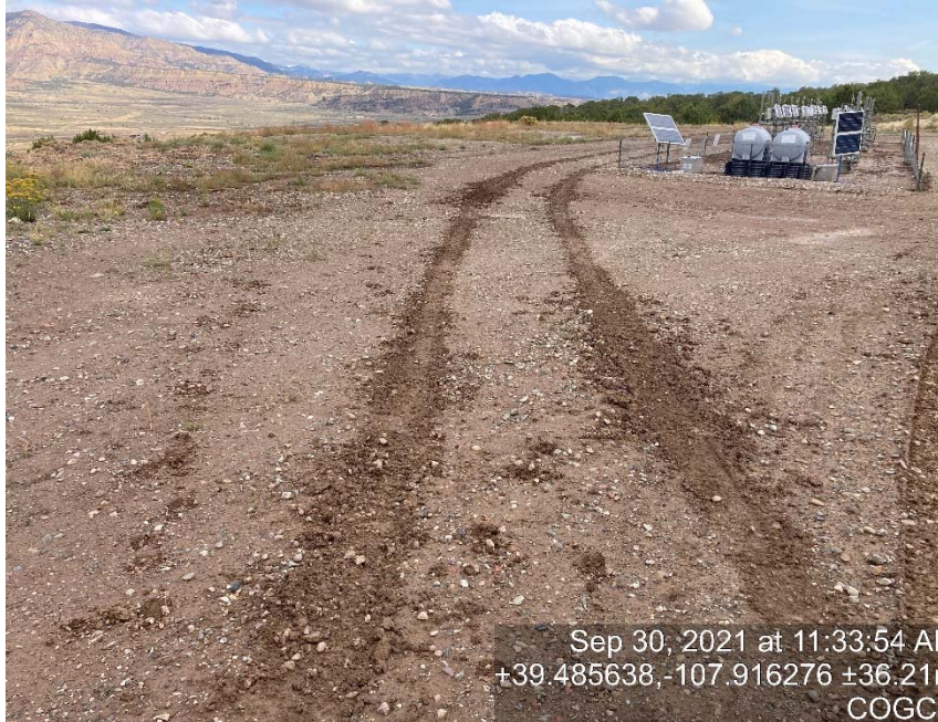
Lack of stabilization/compaction
