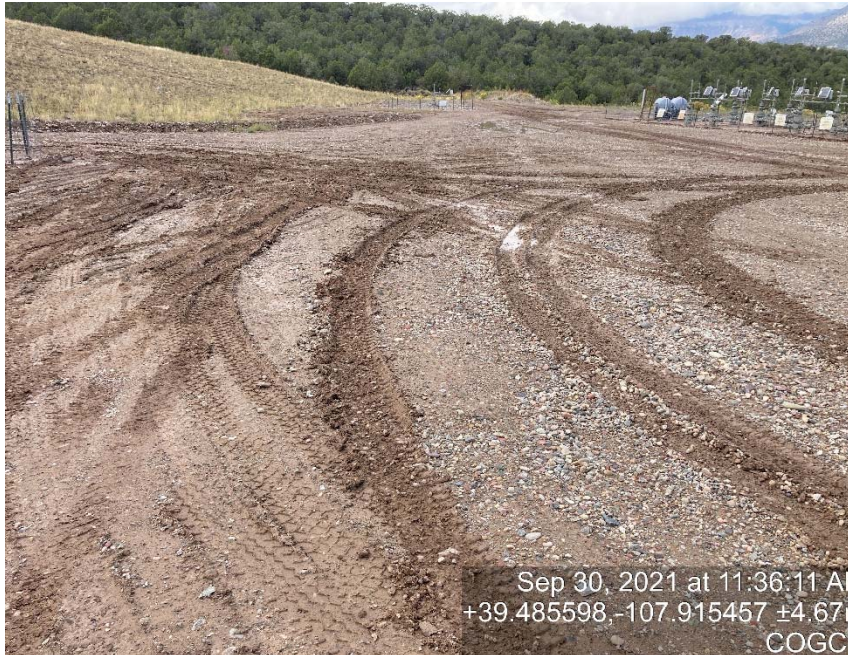
Lack of stabilization/compaction
