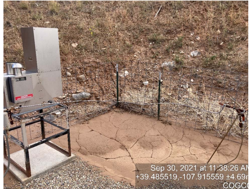
Lack of stabilization/erosion
