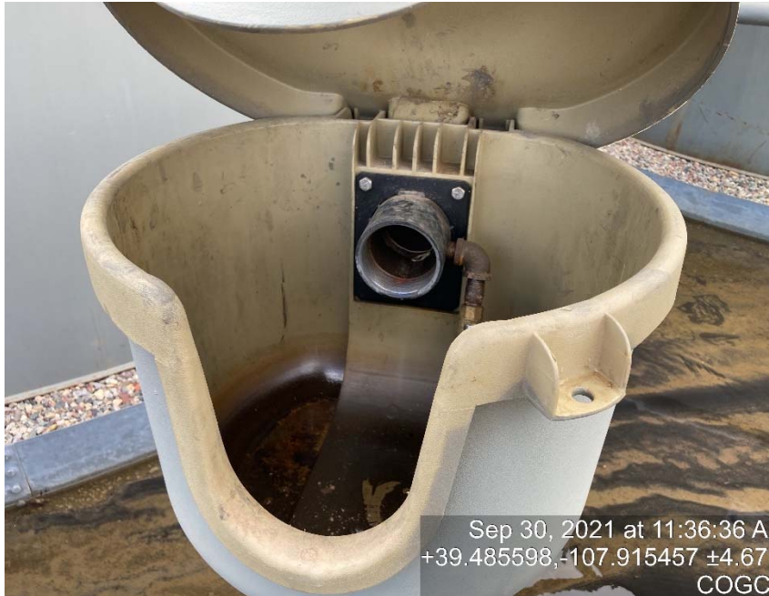
Missing bull plugs/caps on load out lines
