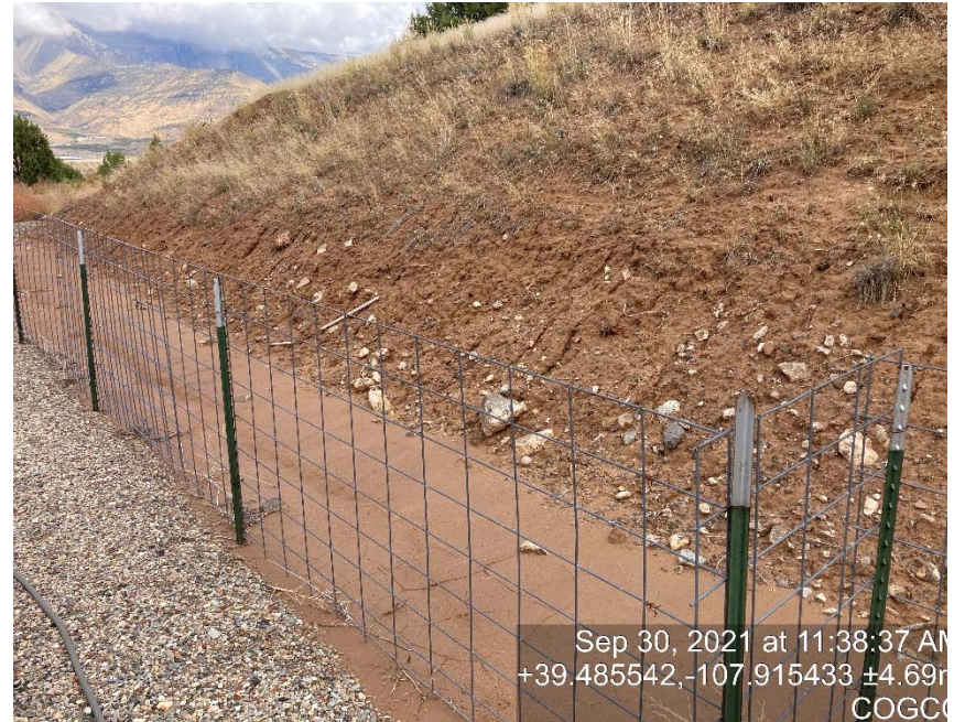
Lack of stabilization/erosion
