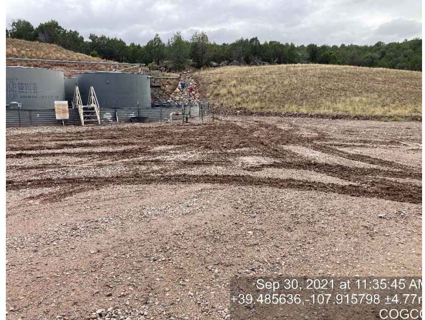
Lack of stabilization/compaction
