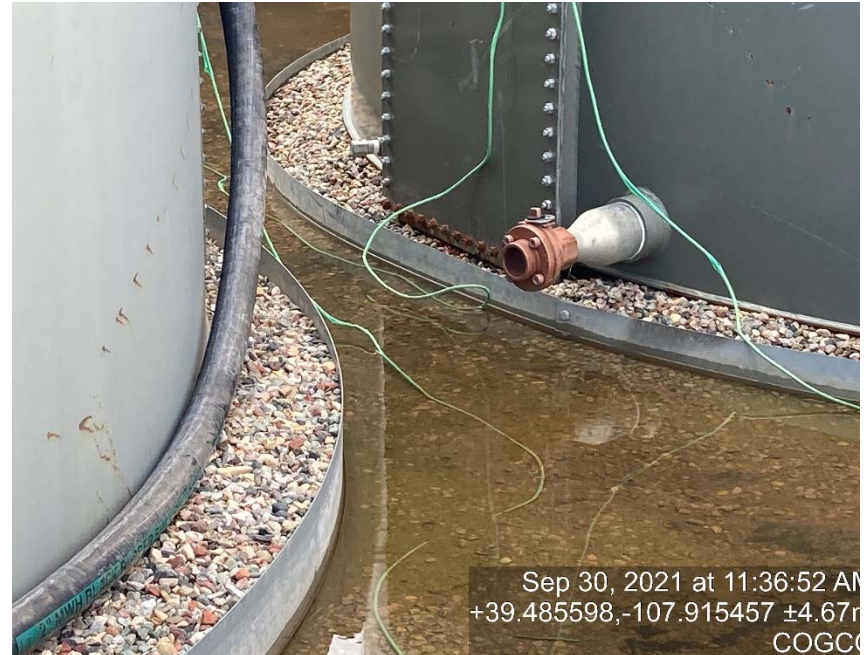
Missing bull plugs/caps on load out lines
