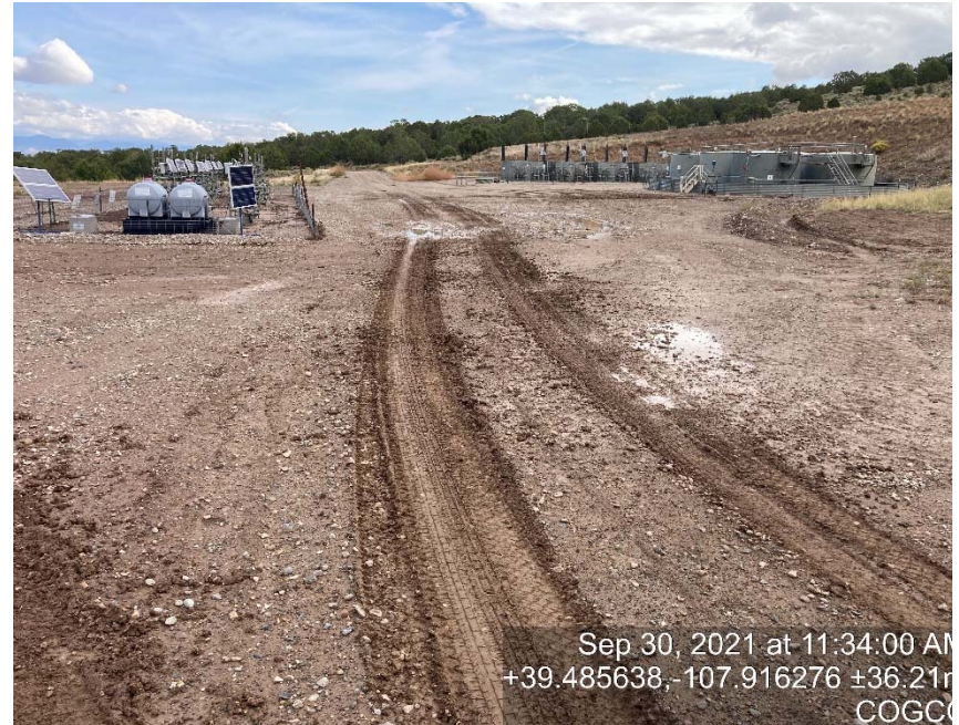
Lack of stabilization/compaction
