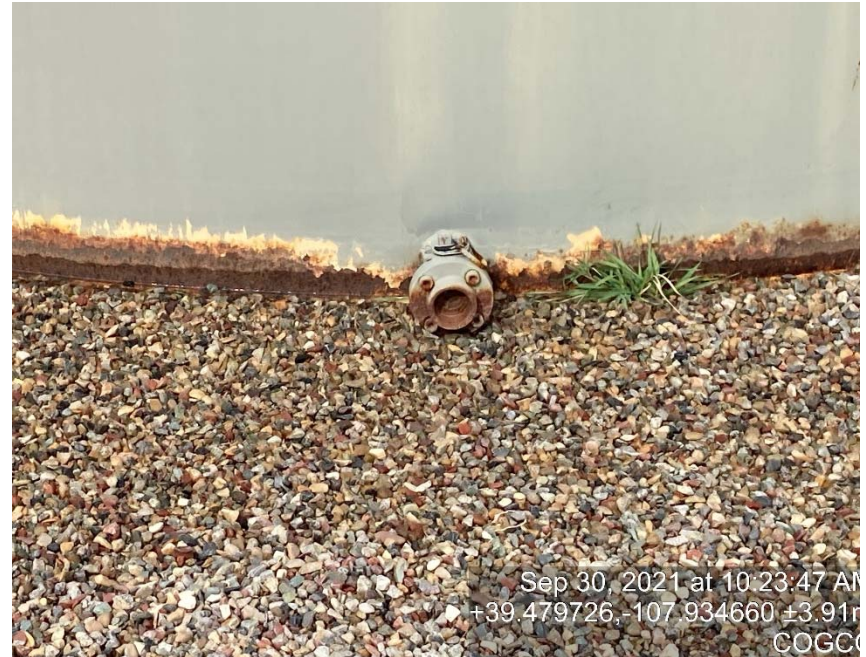
Missing bull plug/caps on load out lines
