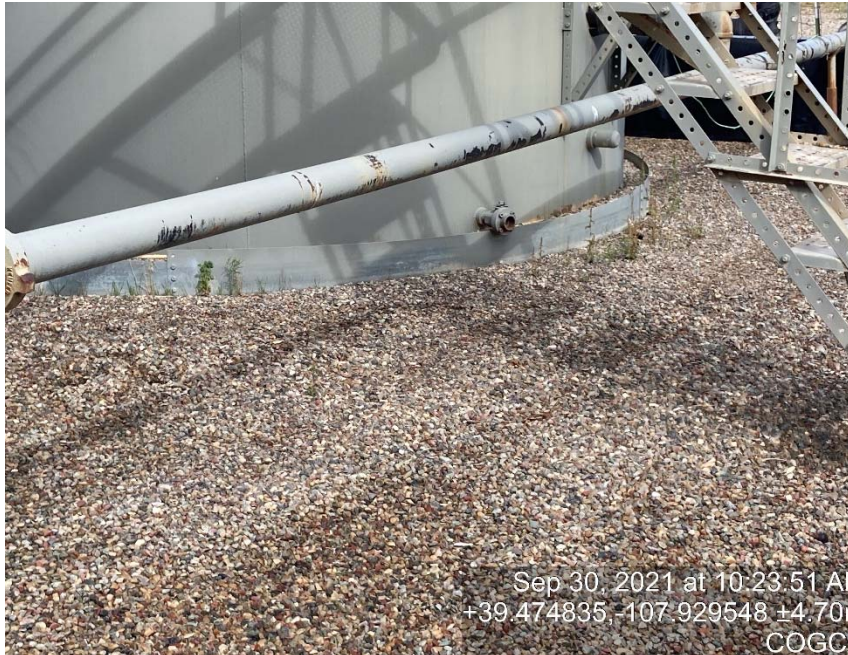
Missing bull plug/caps on load out lines
