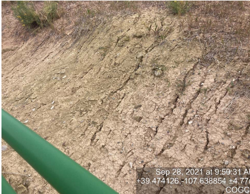
Lack of stabilization/erosion
