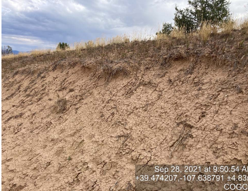
Lack of stabilization/erosion
