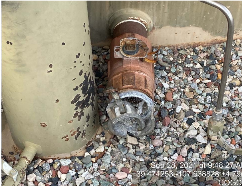
Lack of bull plug/cap and is broken
