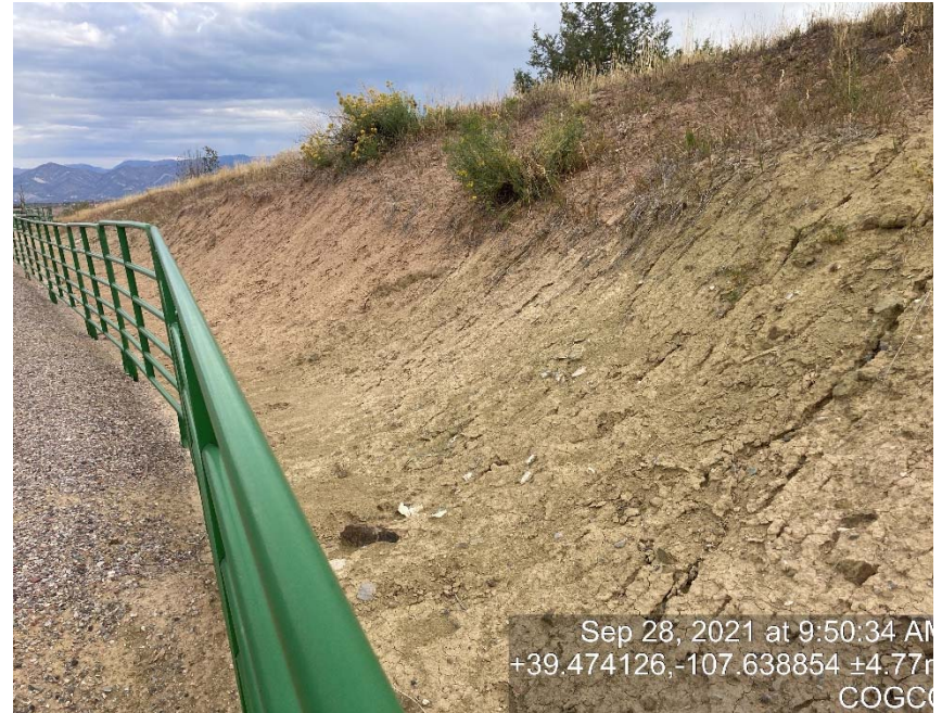
Lack of stabilization/erosion
