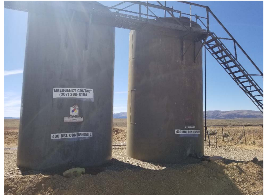
Photo 6. Incomplete tank labels.
