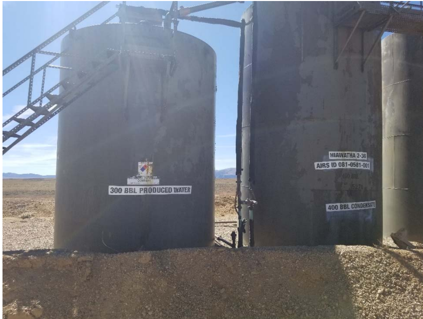
Photo 5. Incomplete tank labels.
