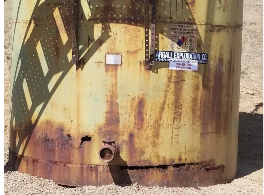
Photo 3. Close up of photo 2 and tank holes. Tank has become debris and must be removed.
