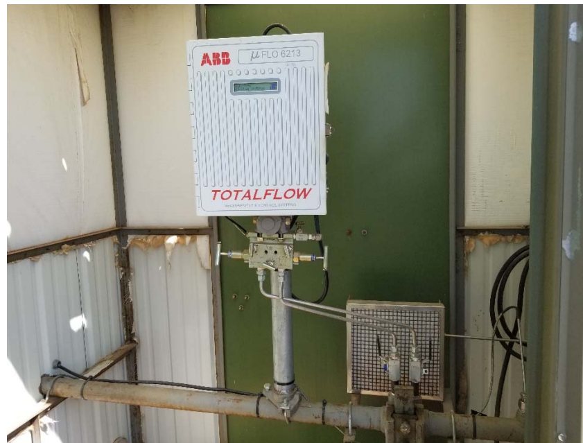
Photo 3. No calibration in gas meter run.
