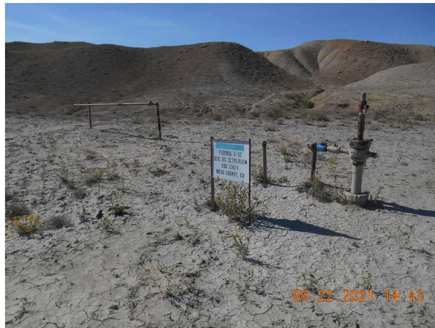
Wellhead with sign. 4-2" flowline risers
