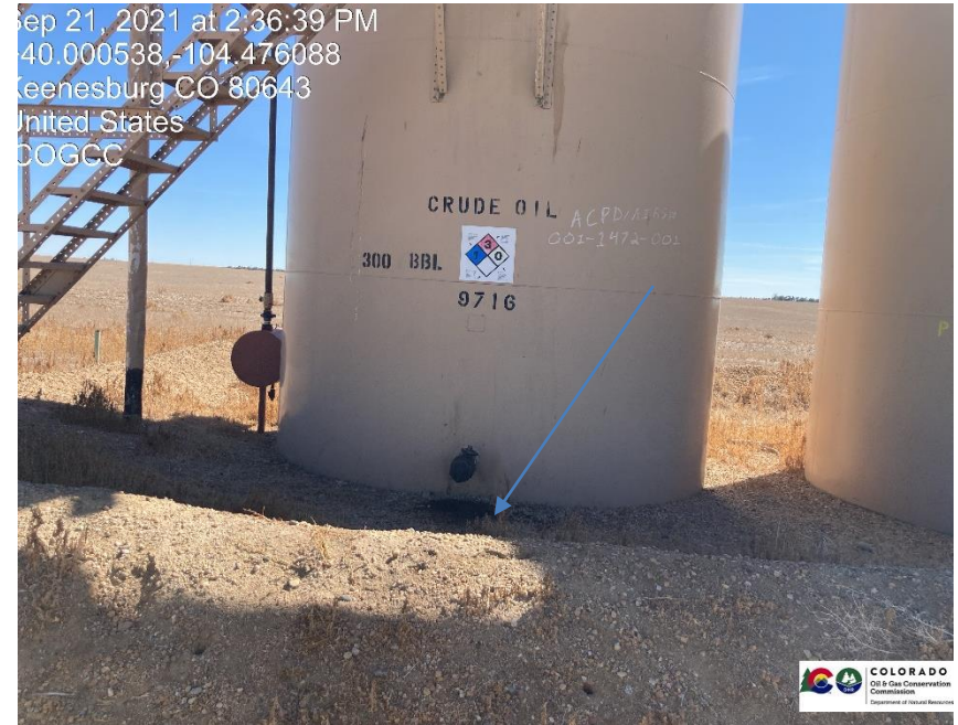
Pic 6 stained soil under loadout valve.
