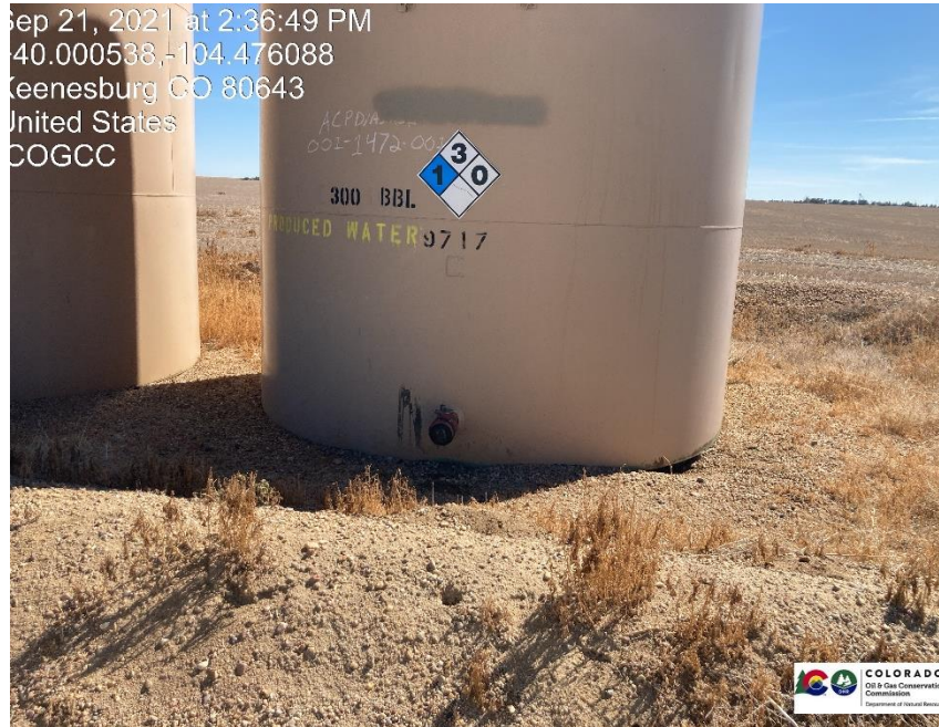
Pic 7 stained soil under loadout line.
