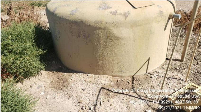
**Photo 15 Stained soil around PW tank**
