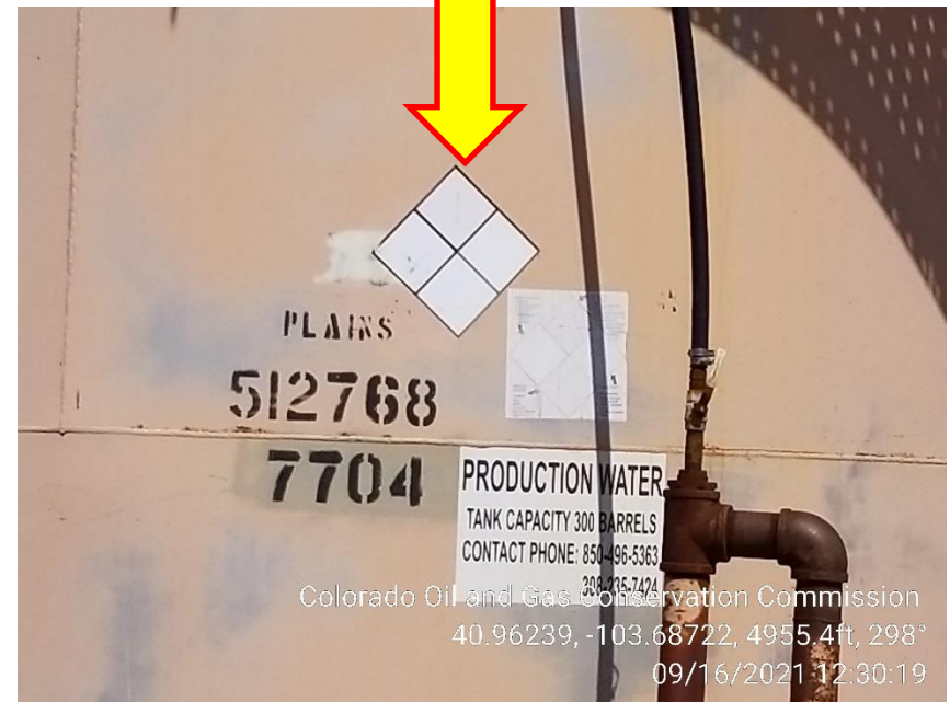
Photo 4 – NFPA Label has faded no longer visible
