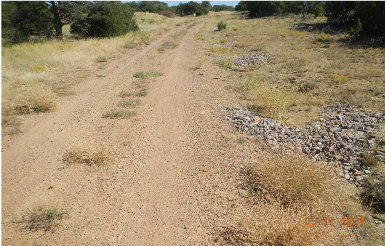
Photo 2. Facing southeast further along the access road. The rock check dams along the road side appear to be controlling erosion.
