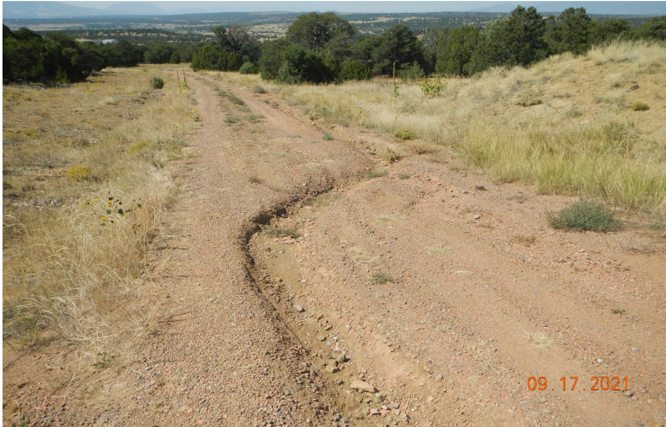
Photo 3. Facing back northwest on the road adjacent to the location. This erosion channel previously observed was never repaired.
