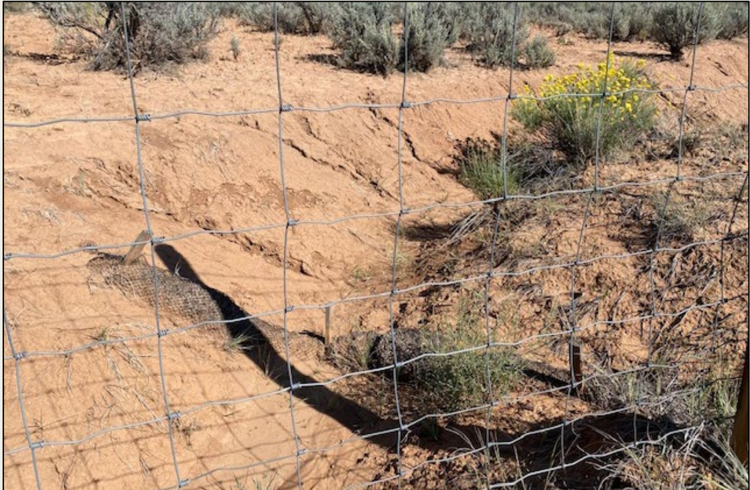
Photo 3. View of erosional channel leading out of the northern edge of the project area, where wattles are inundated, and banks are eroding and lack stabilization. Wattles are not adequate BMPs here.
