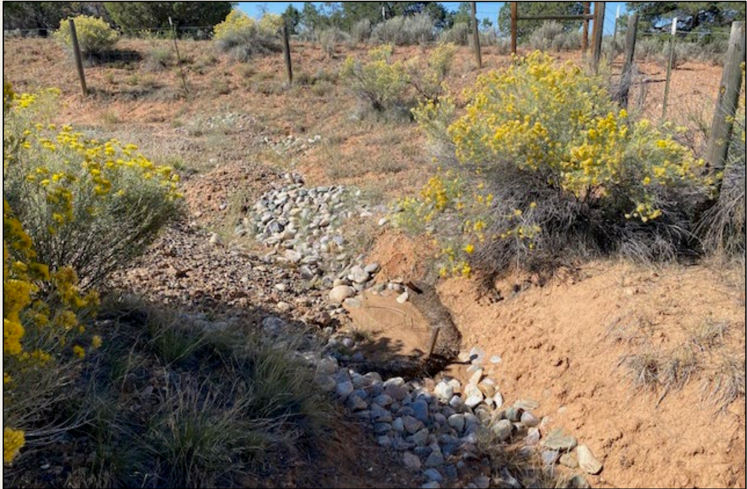
Photo 4. View of area in the northwestern corner of the project area where stormwater flows off of the project area, conveying significant sediment loads and inundating BMPs.
