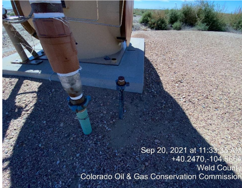
Photo #3 Unmarked/tagged riser
