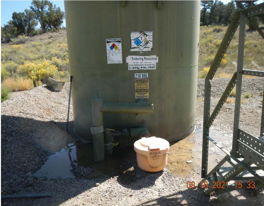
Standing water near base of AST.
