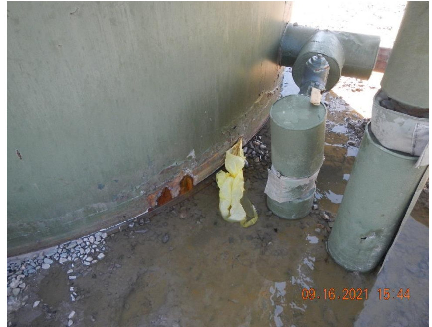
Point source of Spill/Release Point ID #480754 with yellow plastic bag protruding from hole in AST.
