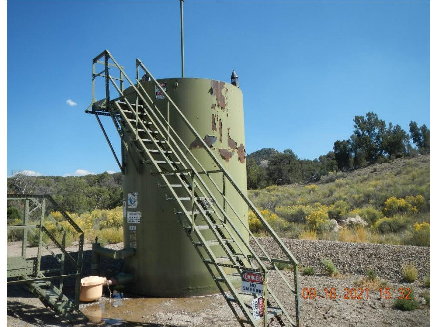
Paint is peeling off of AST. Hole in AST is the point source for Spill/Release Point ID #480754.
