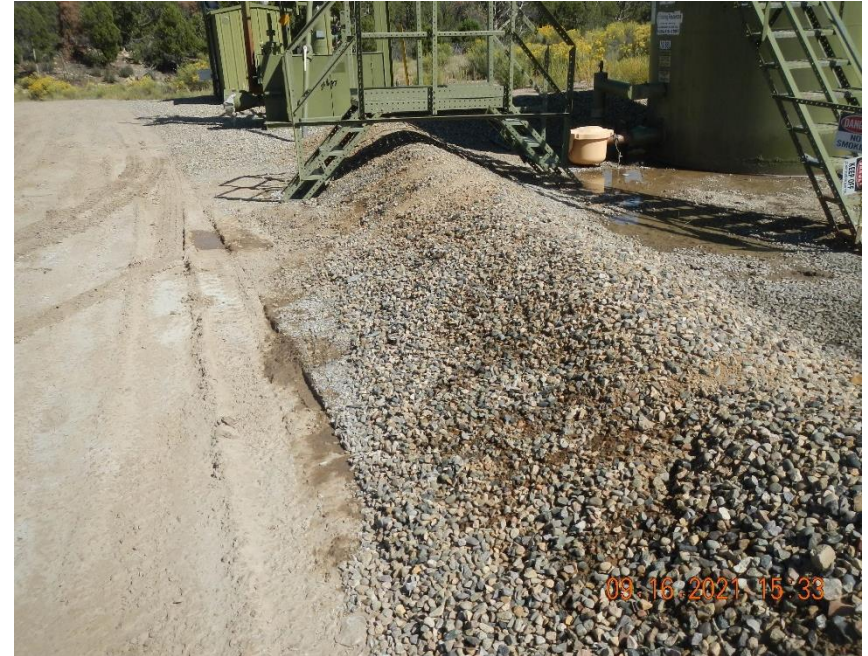
Secondary containment berm is wet and stained.
