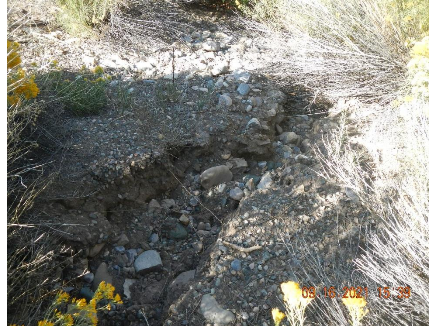
Incised erosional channel on fill slope along northern edge of location.
