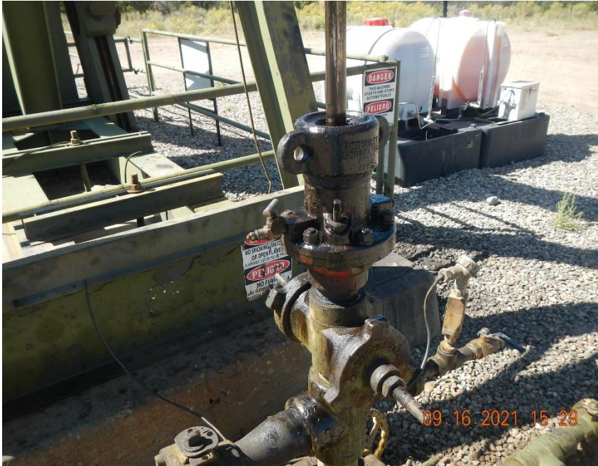
Well head is stained and wet.
