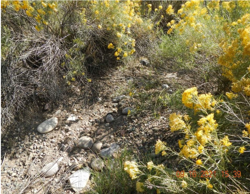
Erosional channel on fill slope along northern edge of location.
