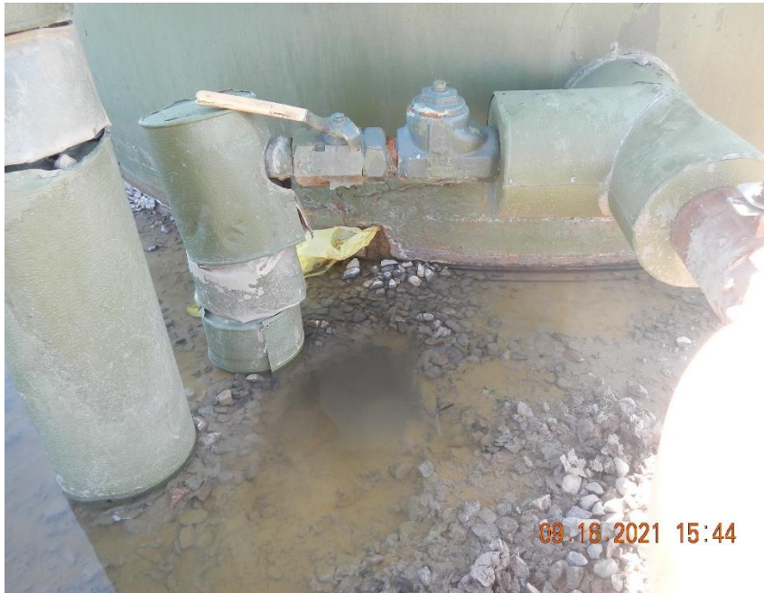
Hole in AST near load out valve. Yellow plastic bag stuck in hole.
