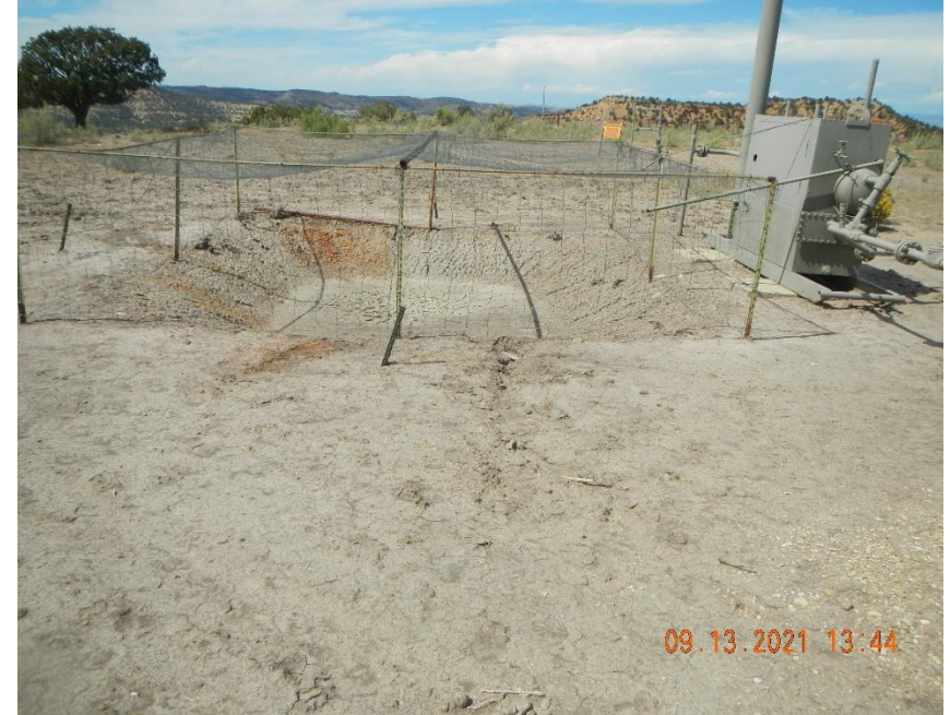
Storm water washing from access road into pit.
