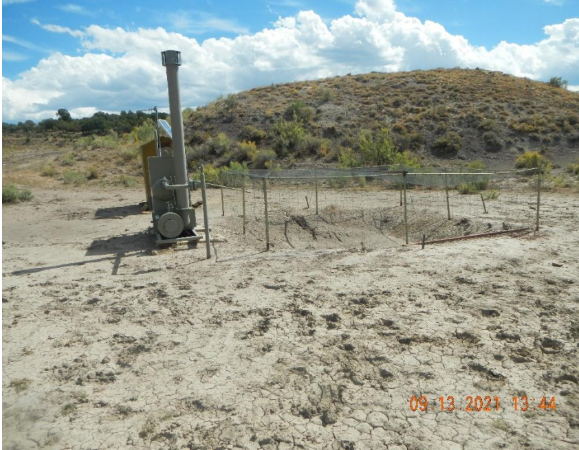
Storm water washing from access road into pit.
