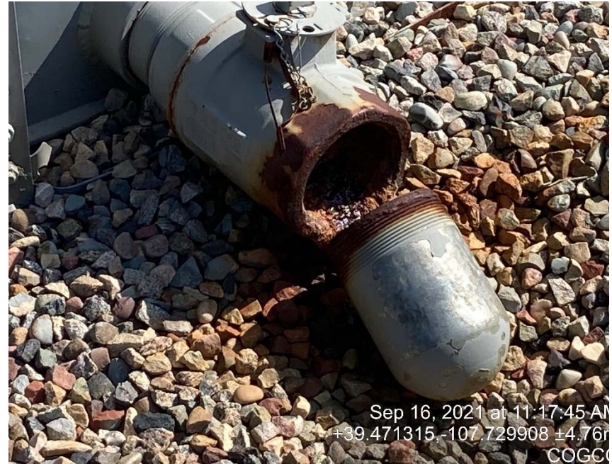
Rusted load out line leaking/cap not installed
