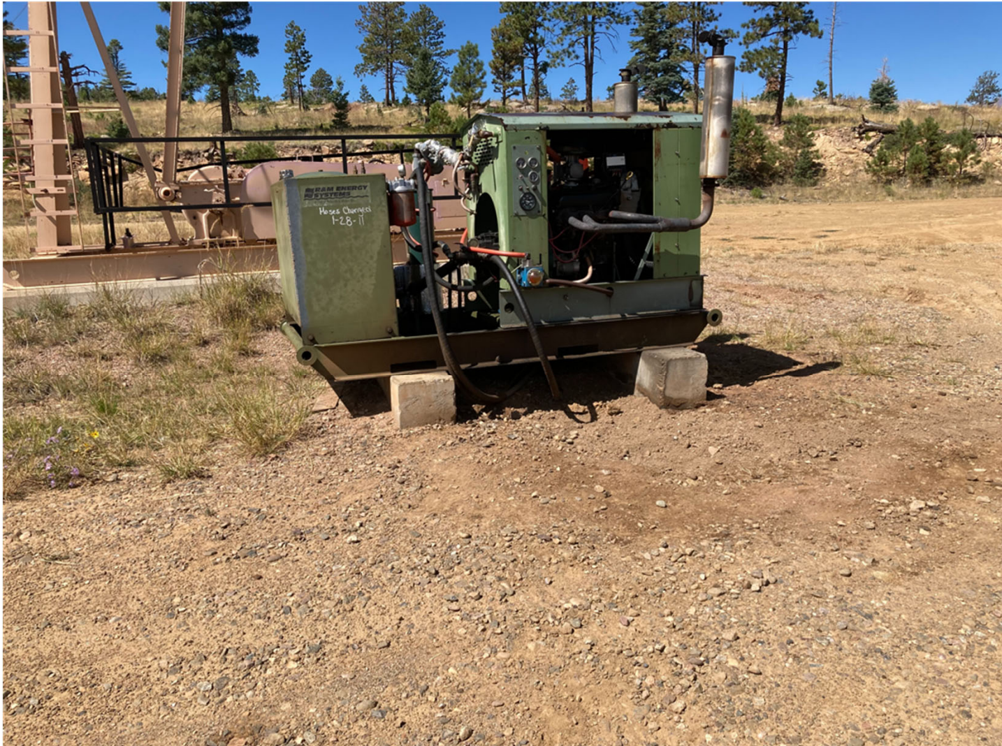
PHOTO 1: MAINTENANCE WAS CONDUCTED TO THE ENGINE SKID. THE IMPACTED SOIL/GRAVEL NEXT TO THE SKID WAS CLEANED UP AND REMOVED FROM THE LOCATION. THE SELF INSPECTION PROCESS WAS REVIEWED
