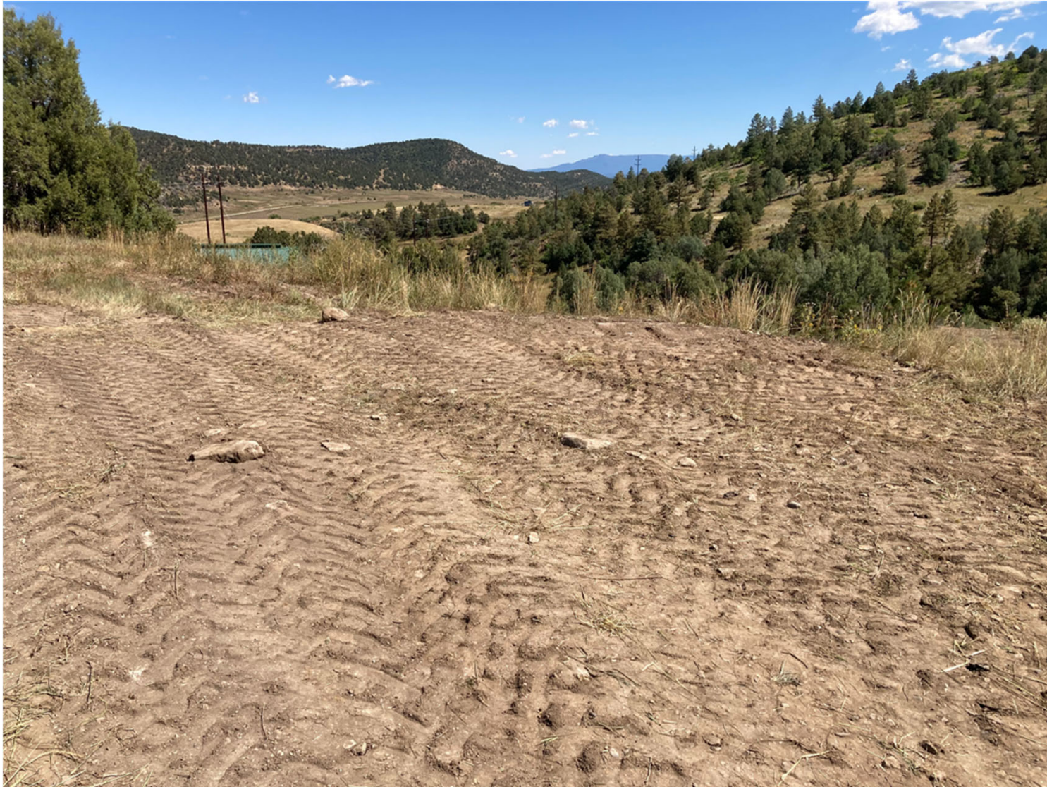
PHOTO 2: THE RISER, POLYPIPE AND VALVE CAN WERE REMOVED FROM THE LOCATION. THE DISTURBED SOIL WAS SEEDED USING THE CPW APPROVED SEED MIX TO PROMOTE THE ESTABLISHMENT OF VEGETATION. THE EXISTING ROOT SYSTEM WAS NOT DISTURBED, VEGETATION SHOULD BEGIN TO EMERGE AFTER PRECIPITATION IS RECEIVED.
