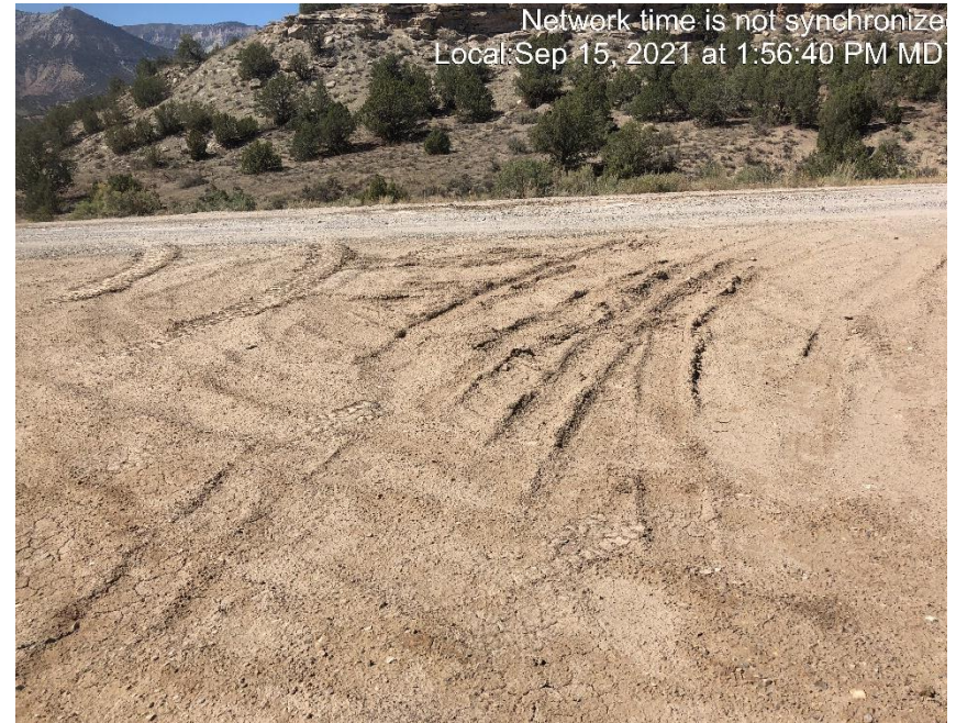
Photo #4895 insufficient tracking control at entrance to location.
