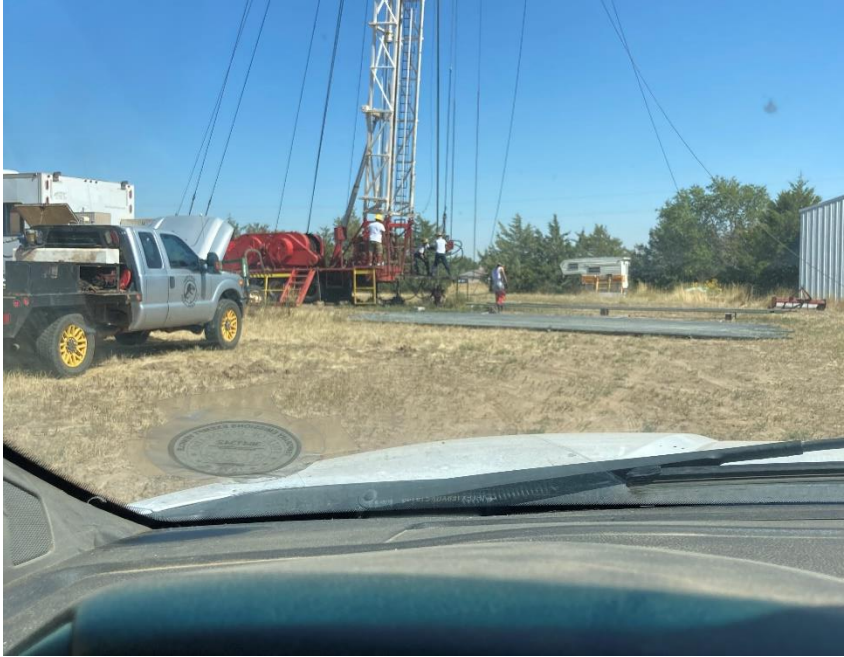
Pic 13 rig crew laying down tubing.
