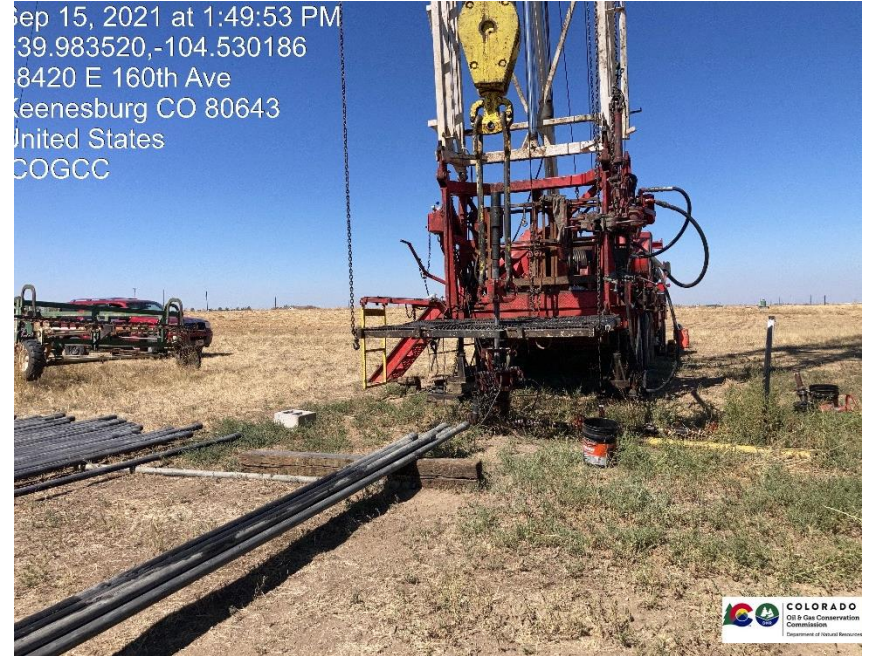
Pic 4 No blow out preventer installed on wellhead
