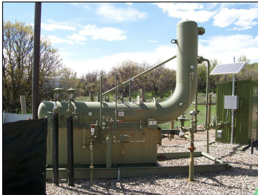
Figure 7 Gravity Separator manufactured by Pesco.
