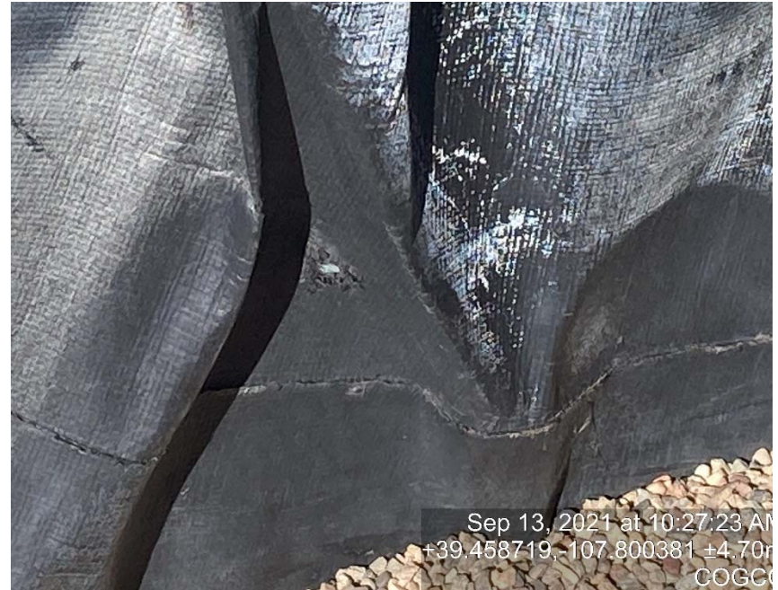
Holes in containment
