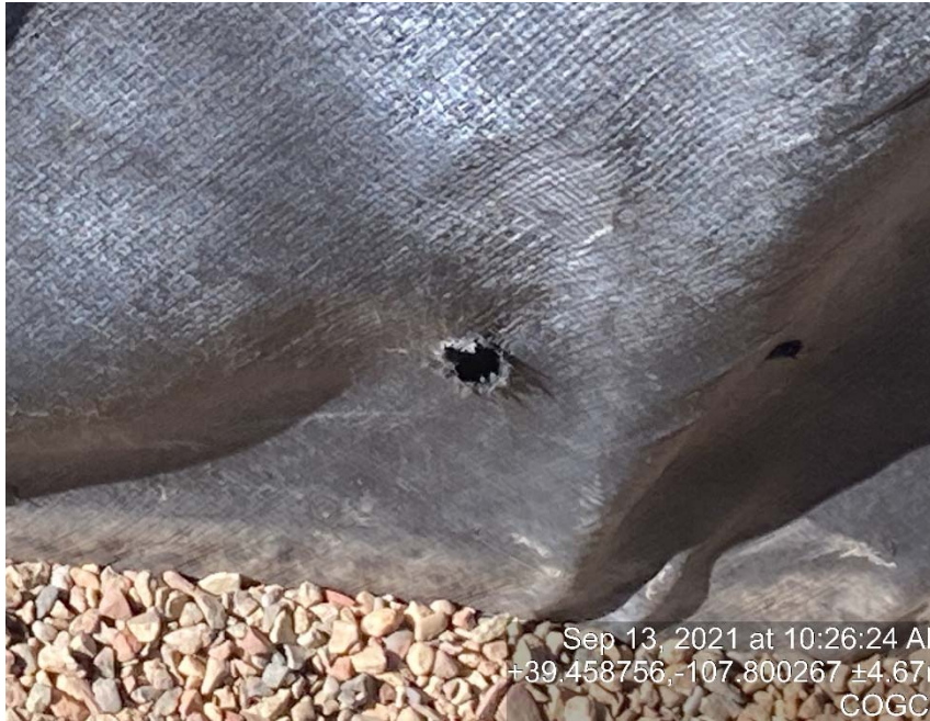
Holes in containment
