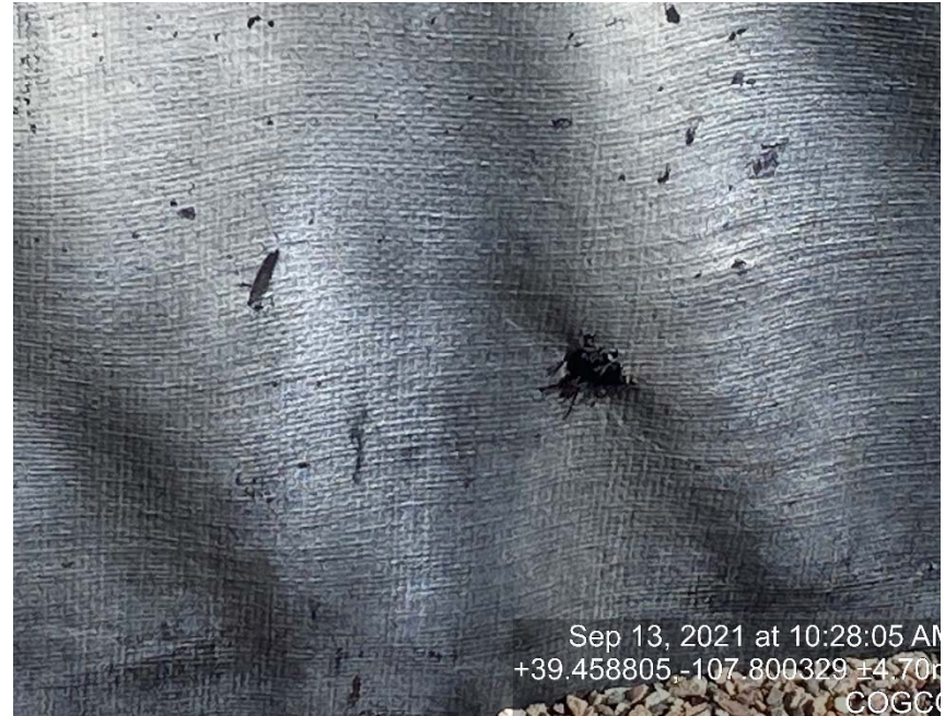
Holes in containment
