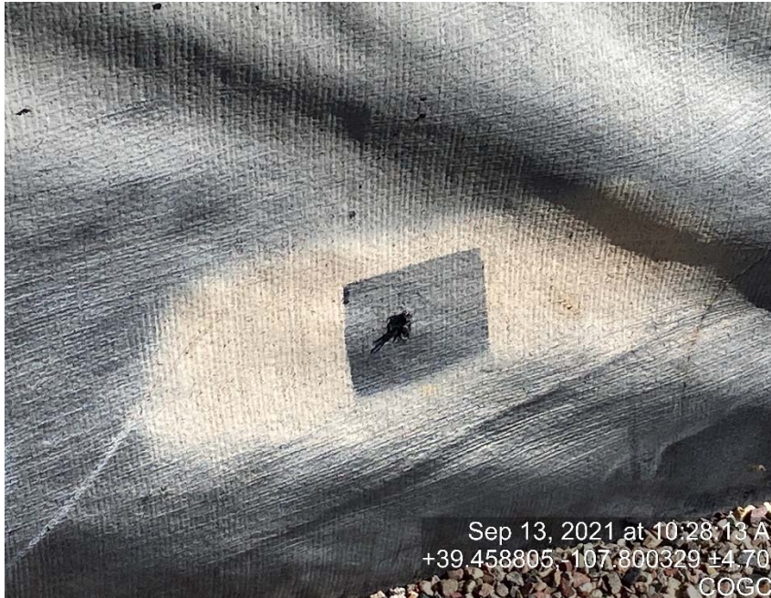
Holes in containment
