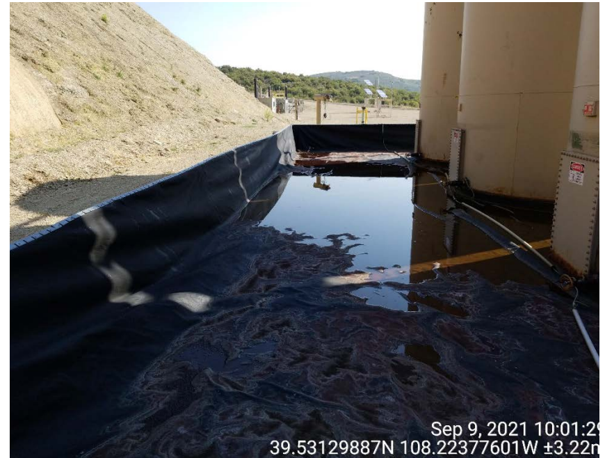
Photo #4 – North side of tank battery secondary containment contained water on inspection date.
