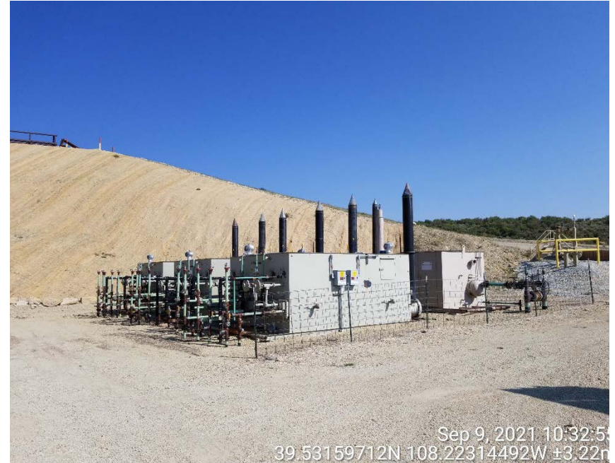
Photo #6 – East bank of separators.
