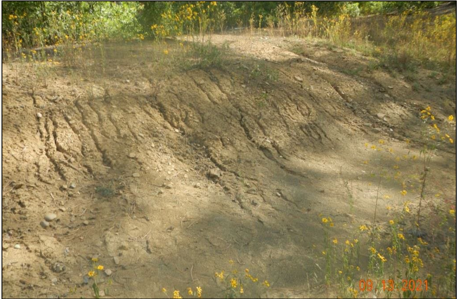
Photo 3. View of rilling erosion occurring within the northern cut-slope.
