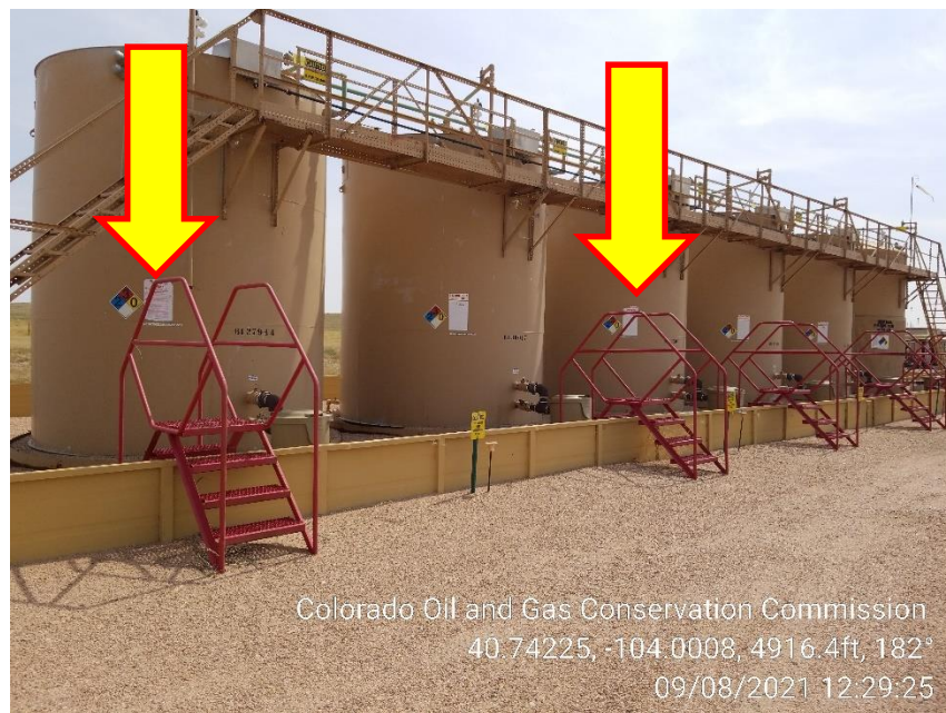
Photo 3 – Tanks STILL missing Capacity Labels. North Tank also missing Contents Label
