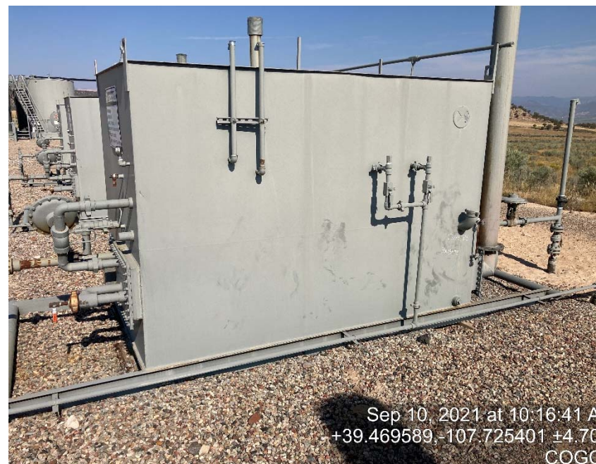
Glycol storage vessels contain no labeling to specify capacity or chemical hazard information.
