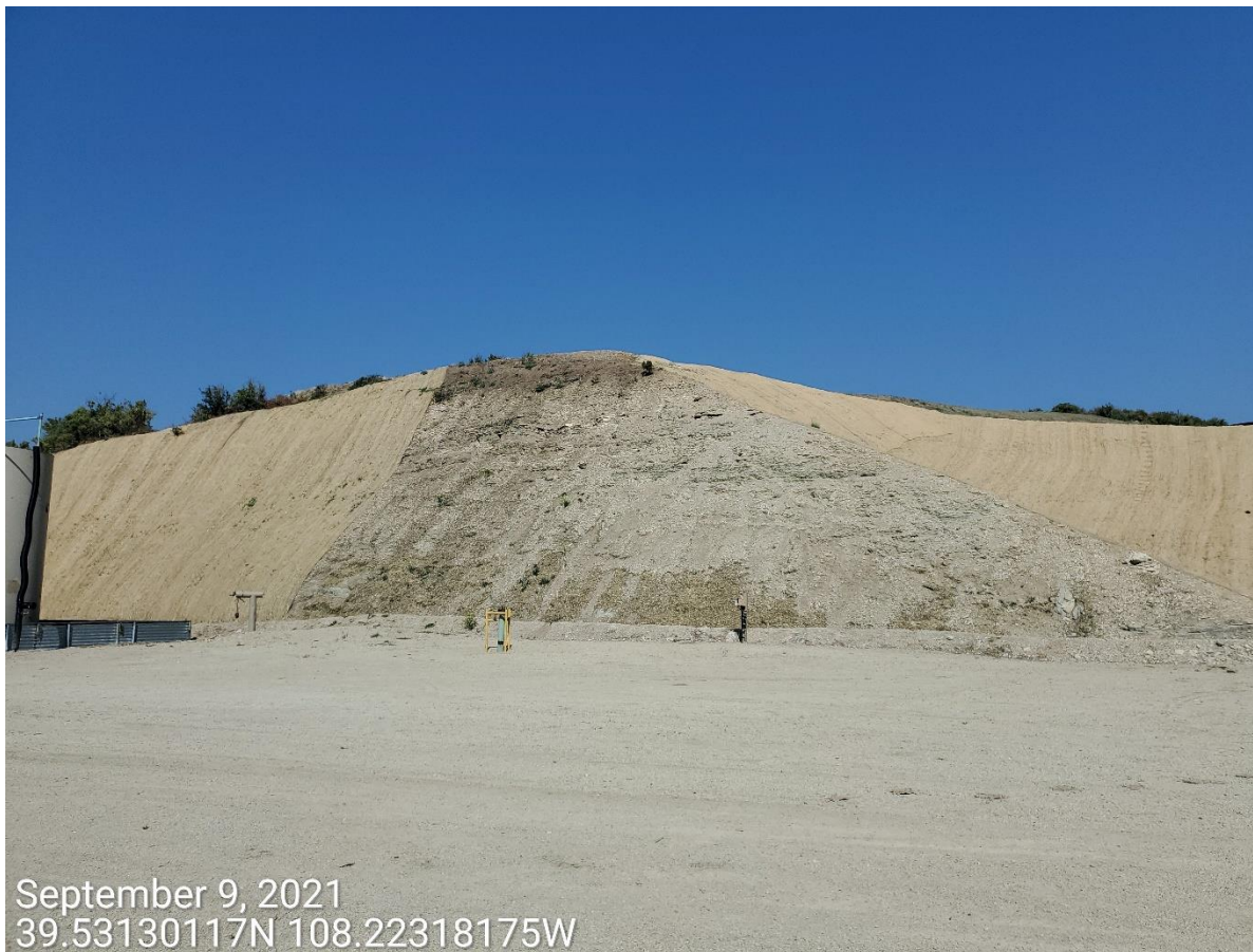
Photo 1: Photo taken from the Location, facing north. Photo shows large areas where BMPs to protect and stabilize the cut slope remains missing or insufficient.
