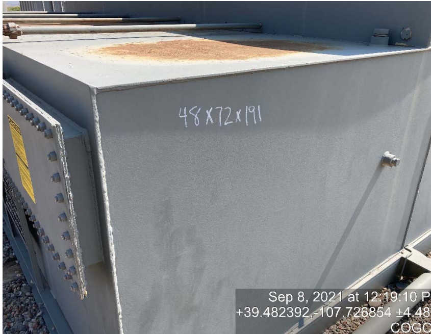
Dimensions of glycol storage vessel
