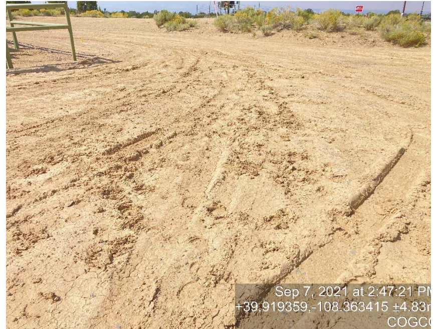
Lack of stabilization/compaction
