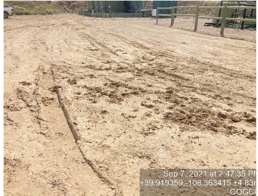
Lack of stabilization/compaction
