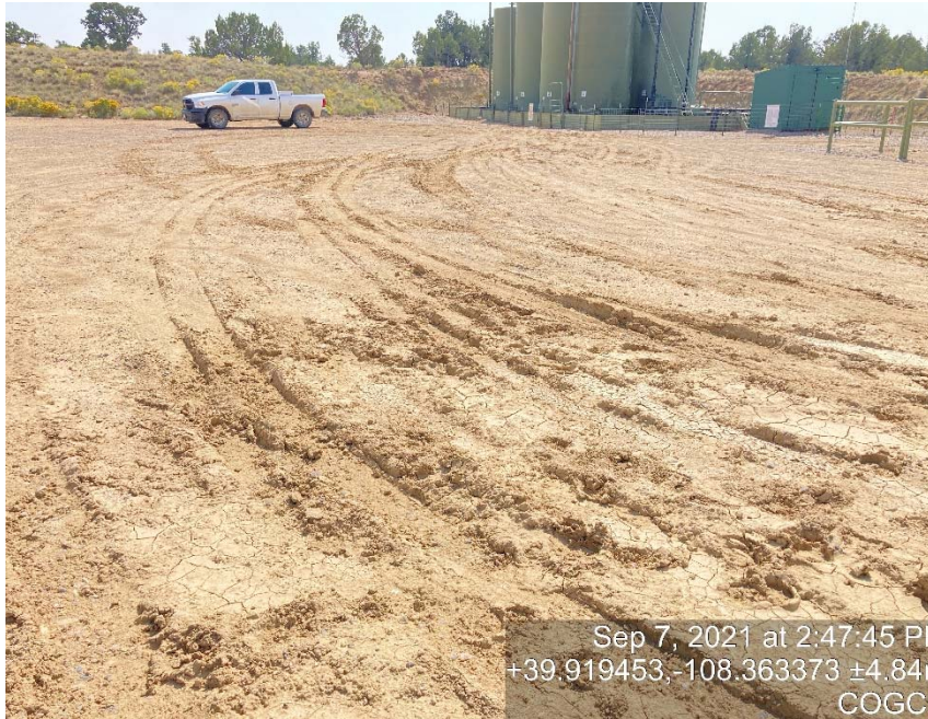
Lack of stabilization/compaction
