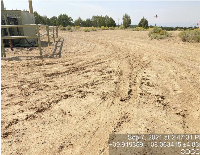
Lack of stabilization/compaction
