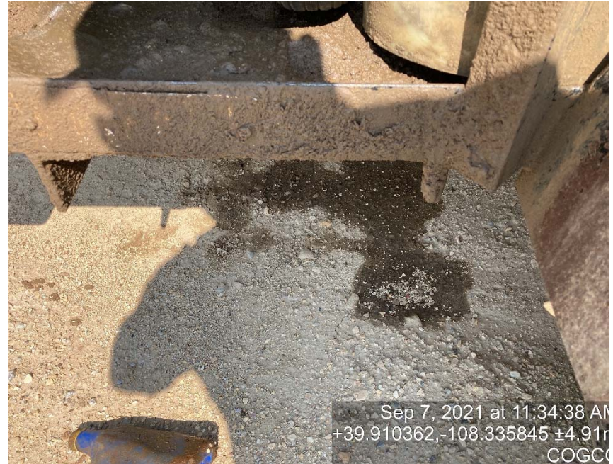
Transfer pump/debris/staining/lack of containment
