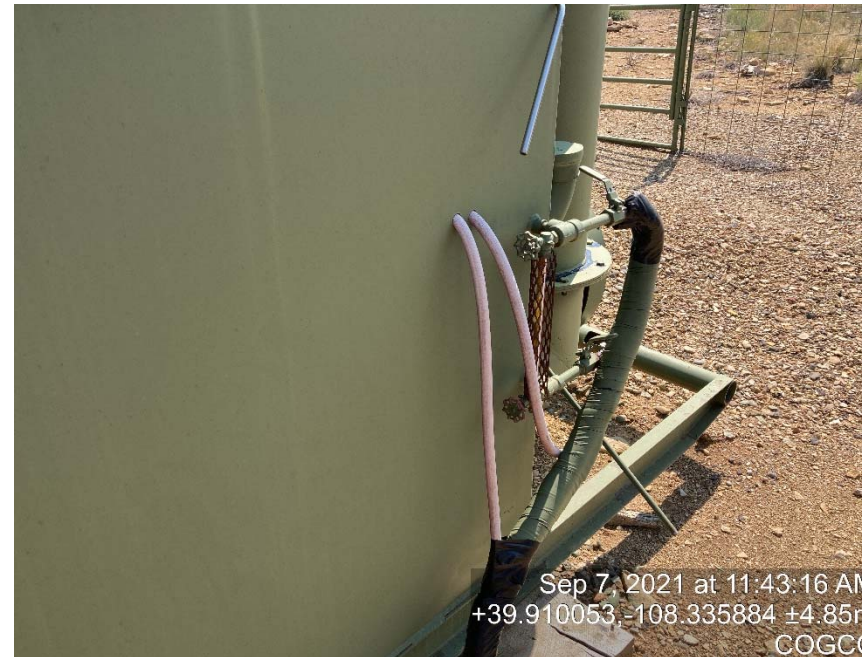
Lack of labeling/glycol pump heat trace lines
