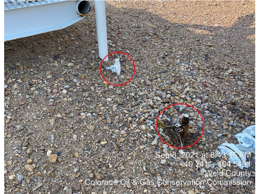
Photo #4 Unmarked, not LO/TO risers.
