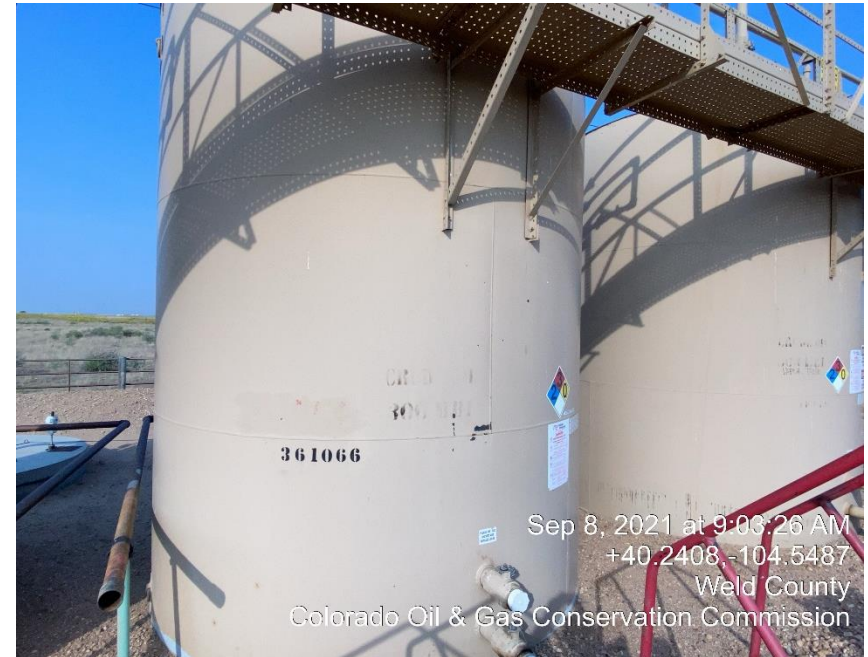
Photo #10 Missing/ Faded Capacity Label
