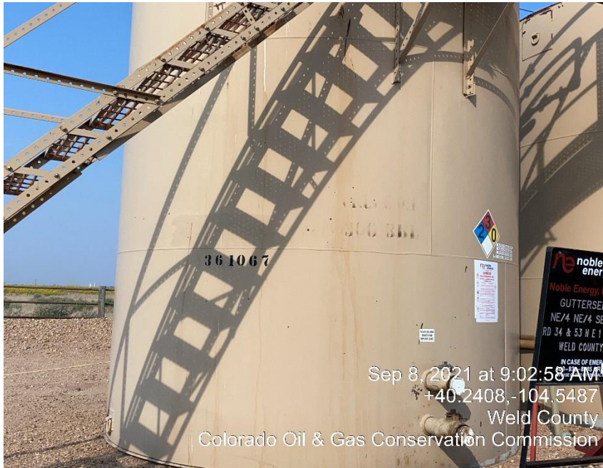
Photo #11 Missing/ Faded Capacity Label
