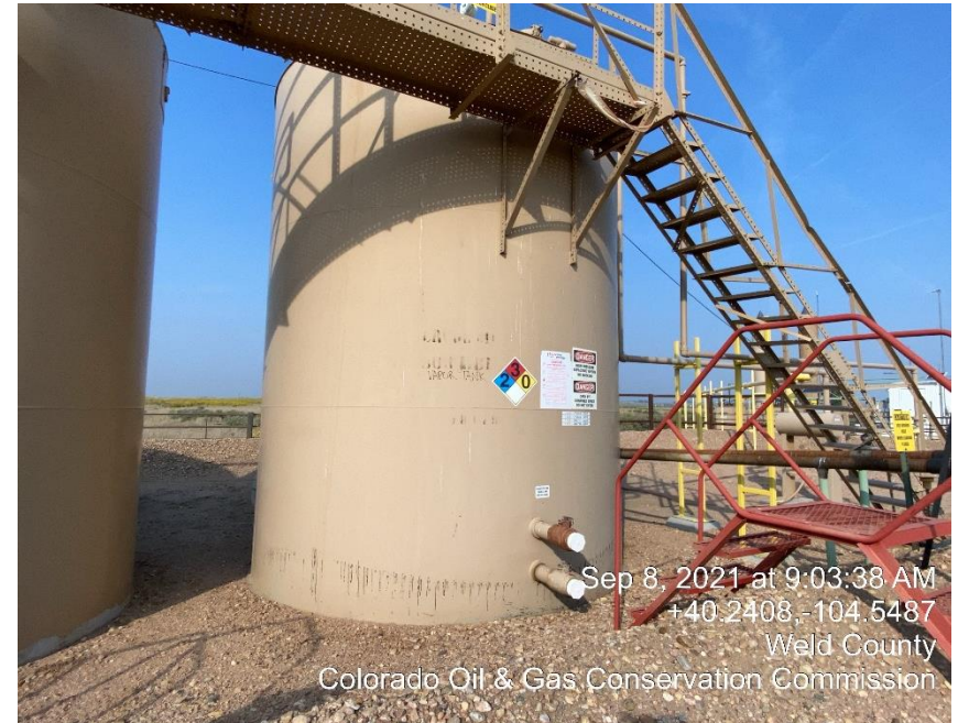
Photo #12 Missing/ Faded Capacity Label
