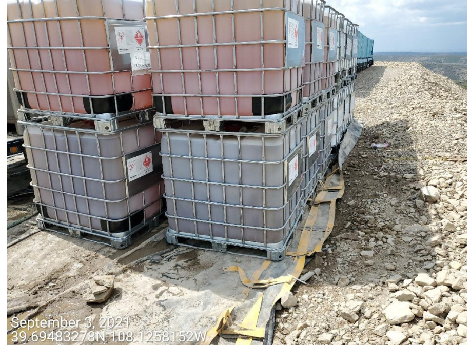
Photo 6: Photo taken from the north end of the Location. Photo shows containment BMP at tanks is not in proper functioning condition to contain a spill.
