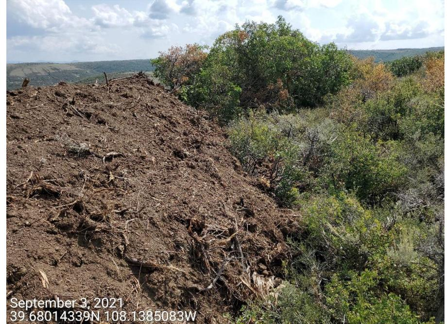
**Photo 6:** Photos provide an example showing BMPs manage runoff, and to protect and stabilize the stockpiled soils are missing of insufficient.
