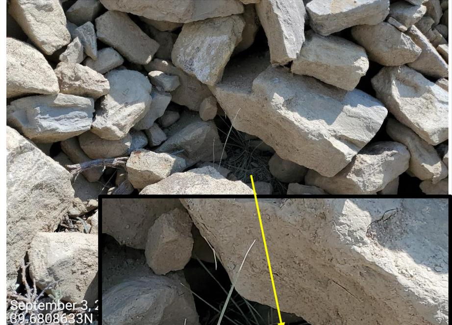
**Photo 4:** Photo taken from the fill slopes on the west end of the Location. Upon removing fill material, Reclamation Specialist was able to observed intact vegetation and topsoil beneath the fill material. Unable to find evidence that Operator properly salvaged, segregated and stored all topsoil within the disturbance area during construction.
