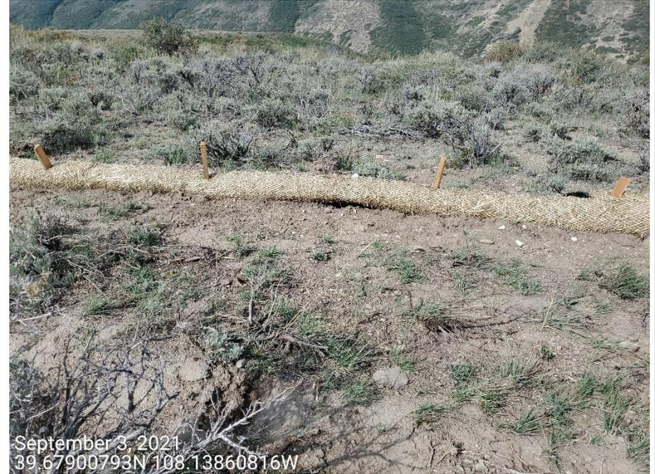
**Photo 2:** Photos provide example of wattle BMPs observed to not be installed in accordance with good engineering practices.
